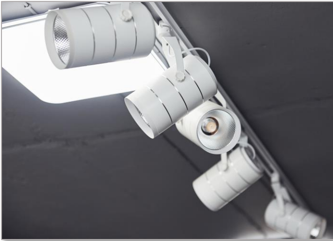
LED lighting and Controls retrofits
