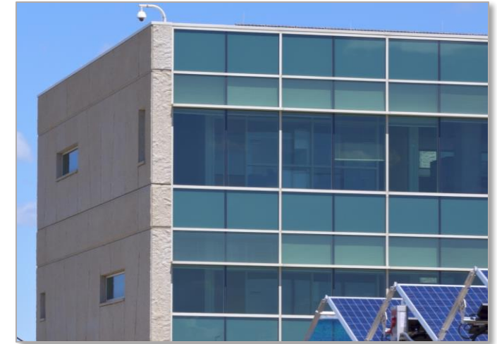
Building envelope improvements and new glazing
