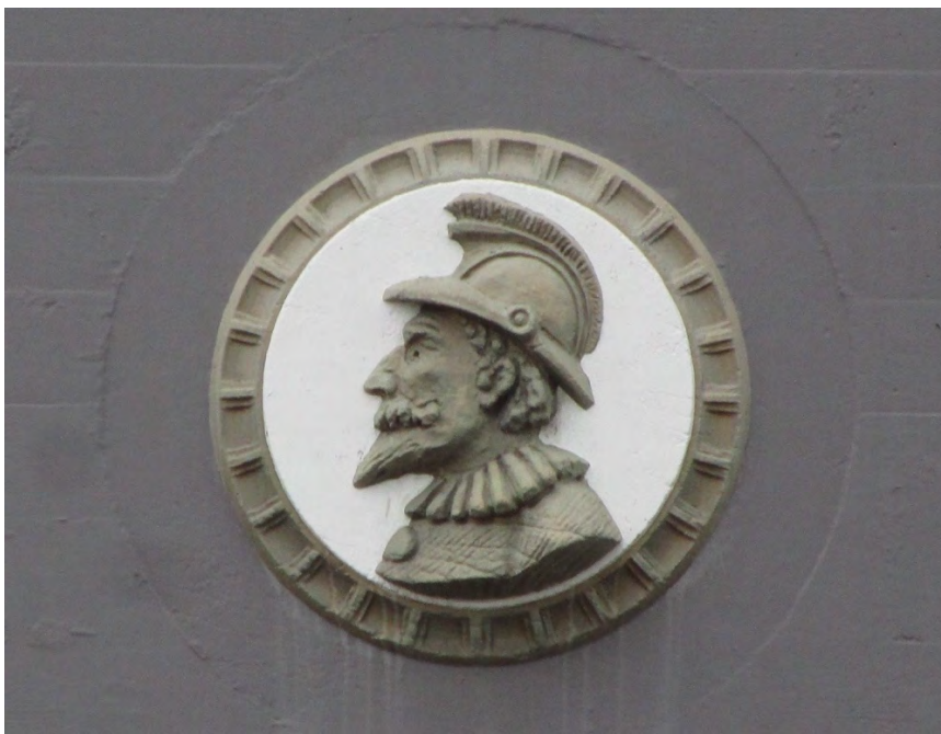
Figure 14: The cast-stone “Spanish Explorer” medallion that will be protected-in-place.
