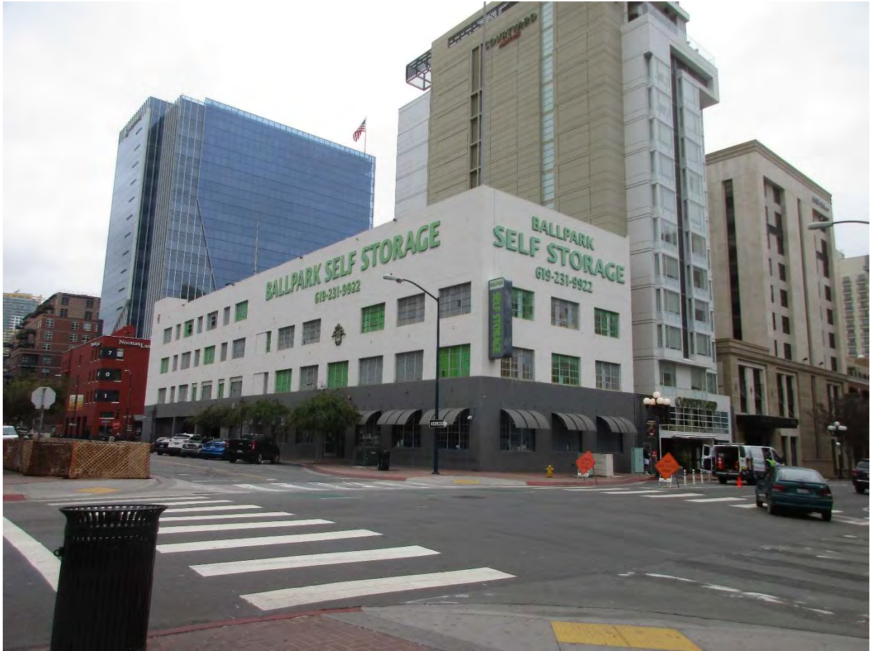
01 LOOKING SOUTHEAST ACROSS ISLAND AVE AND SIXTH STREET INTERSECTION AT THE BALLPARK STORAGE BUILDING.
