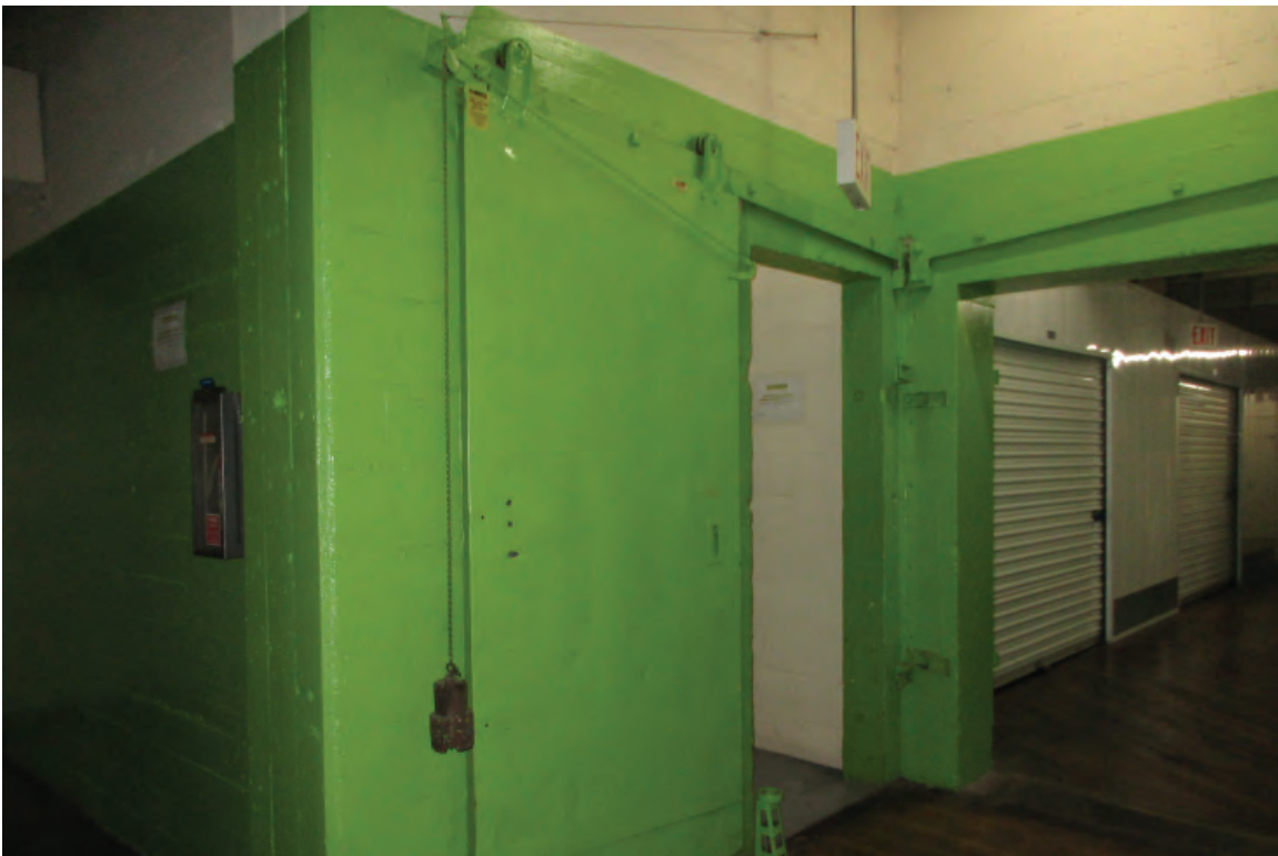
Figure 3-19: View looking northeast at the north stairwell fire door.
