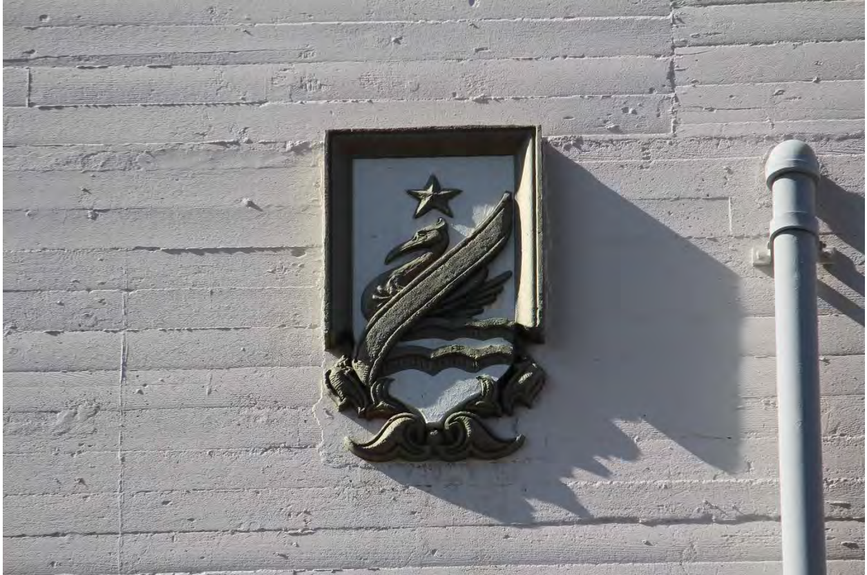
10 DETAIL PHOTO SHOWING ONE OF THE CAST STONE DECORATIVE SHIELDS AT THE EAST ELEVATION.
