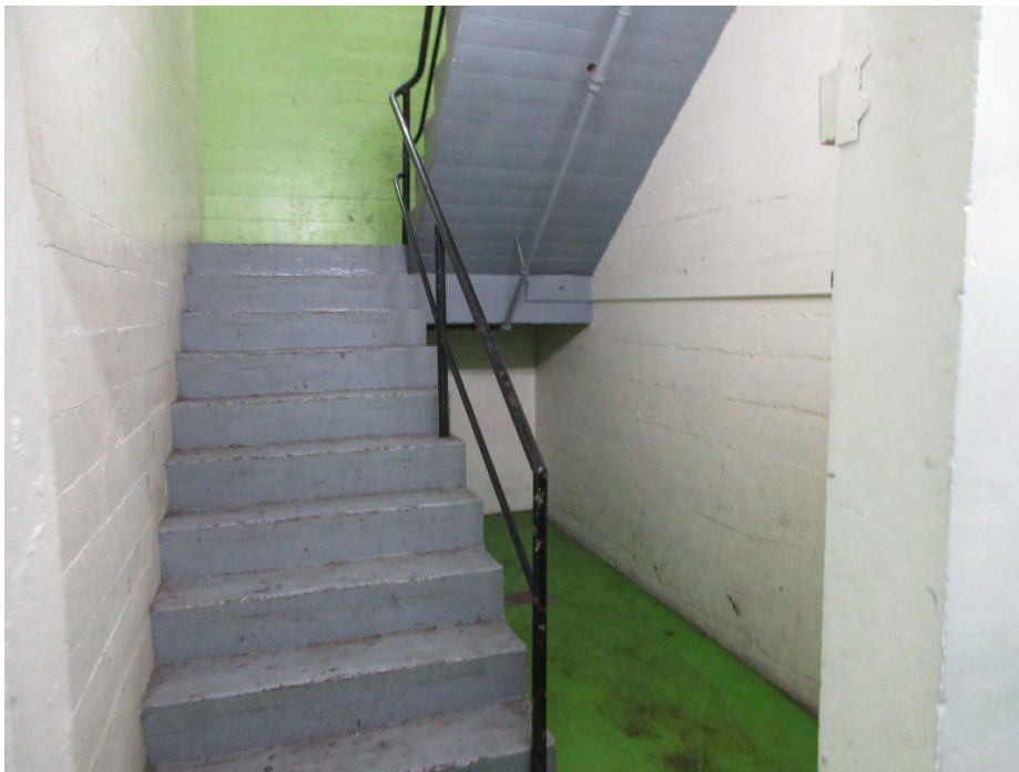
Figure 20: Interior view showing an original concrete stair with steel pipe railings. The stairs will be removed.
