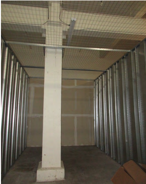
Figure 19: Interior view showing a typical storage space and original post and beam construction. These will be removed.
