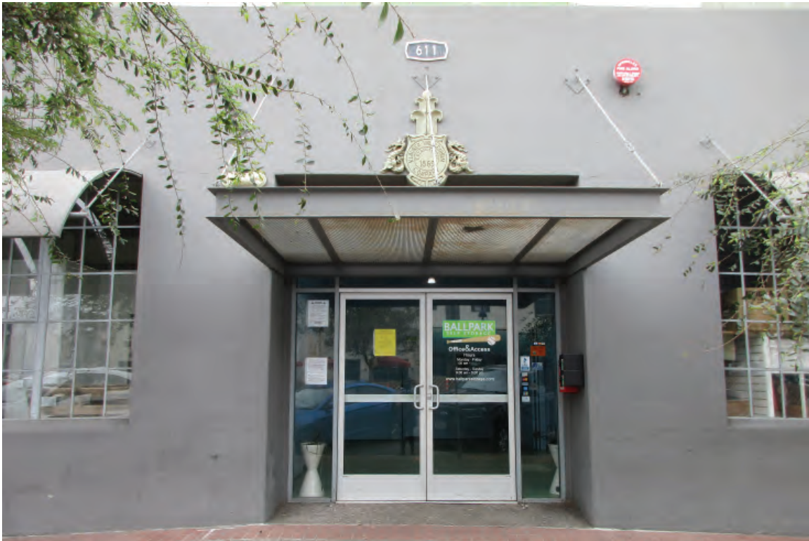
Figure 3-6: Looking south at the primary entrance at the north façade. The primary entry consists of contemporary aluminum storefront doors and window system.
