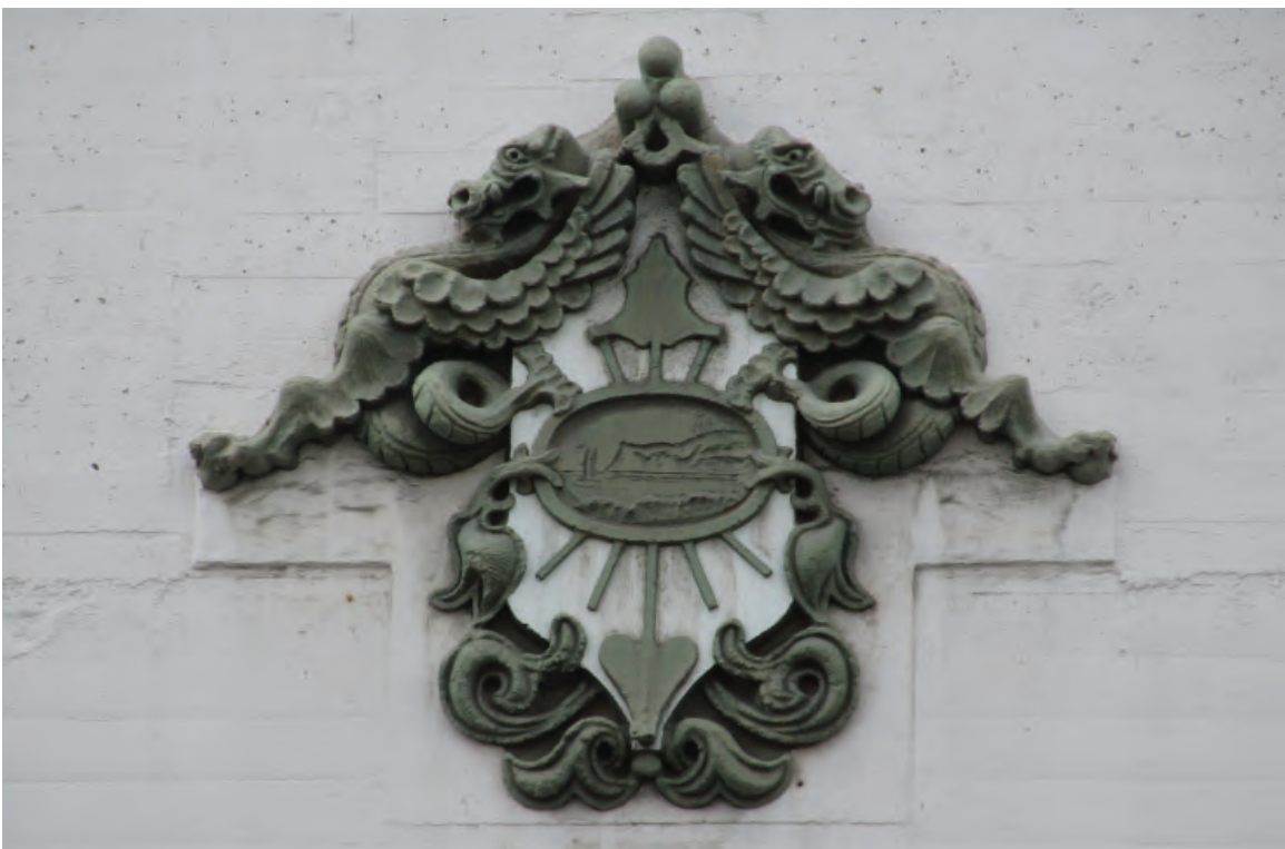
Figure 3-9: Decorative cast-stone shield located above the main entry at the third floor north façade.
