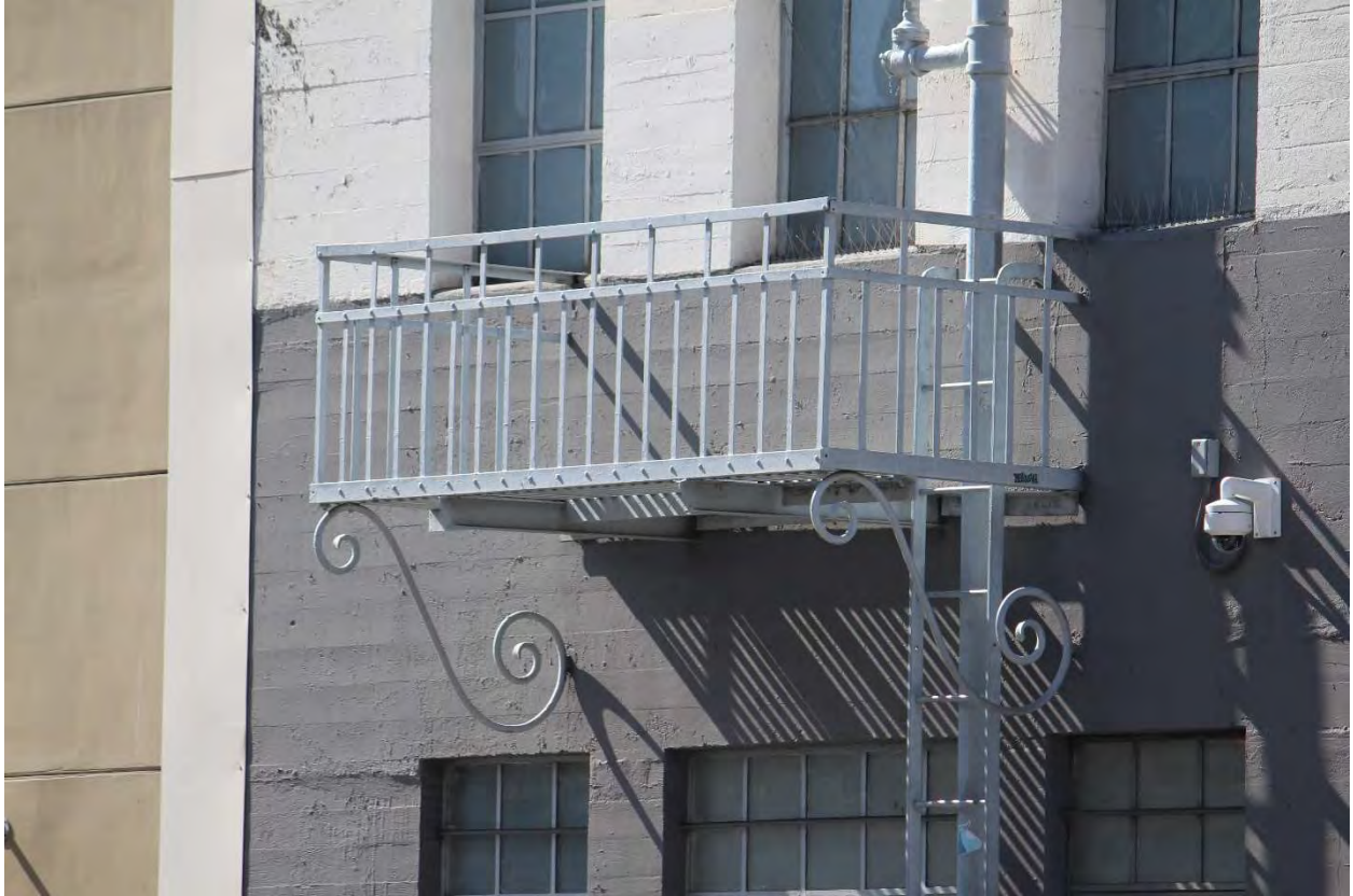
11 ORIGINAL STEEL FIRE-ESCAPE BALCONY AT THE SOUTHERN END OF THE EAST FACADE.
