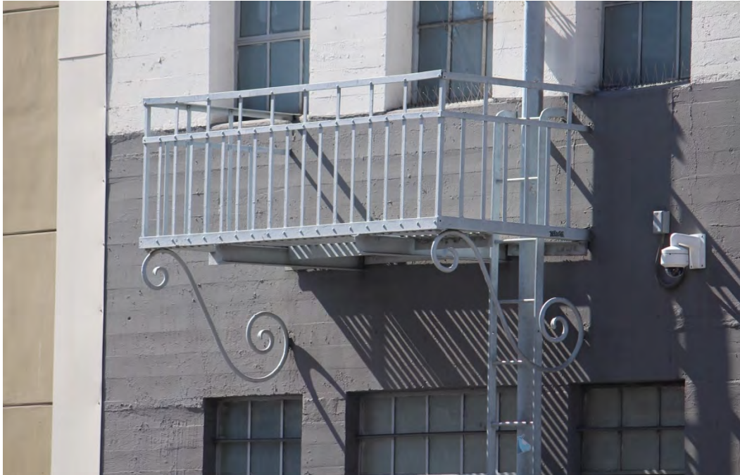
Figure 17: One of two fire escape balconies on the east facade with scrolled bracket supports. These will be incorporated into the rehabilitated facade.
