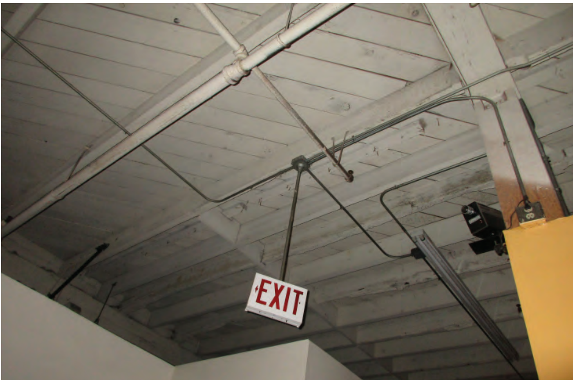
Figure 3-17: Fourth floor west wing looking southwest at the roof framing.
