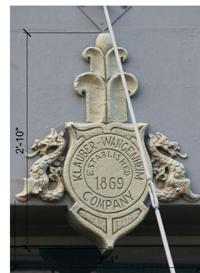
COMPANY SHIELD ABOVE MAIN ENTRY (FIRST FLOOR - NORTH ELEVATION)
