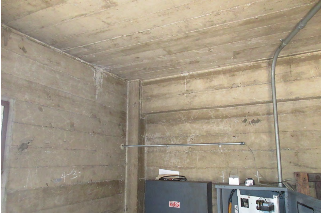
Figure 7: View of the interior of an elevator equipment room on the roof where the original yellow/beige integral concrete color is exposed. Aside from soiling, this is the original color of the building's exterior walls.
