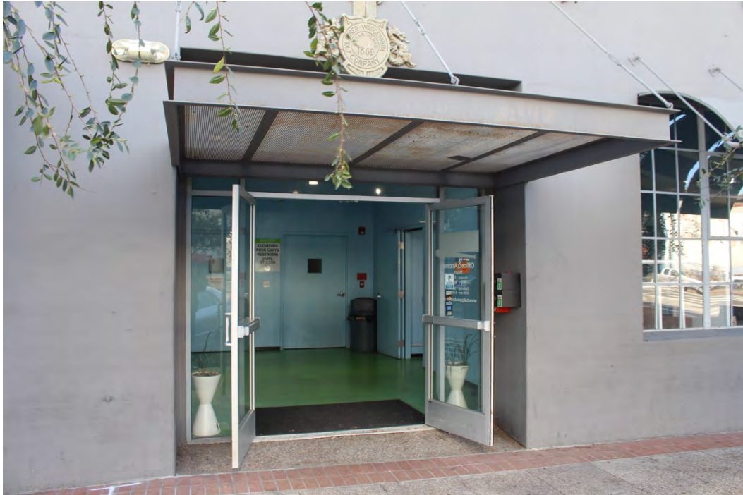
Figure 9: The main entry at the north facade has non-historic aluminum doors and transoms. The steel canopy is also contemporary. The shield above is historic (see Figure 13).
