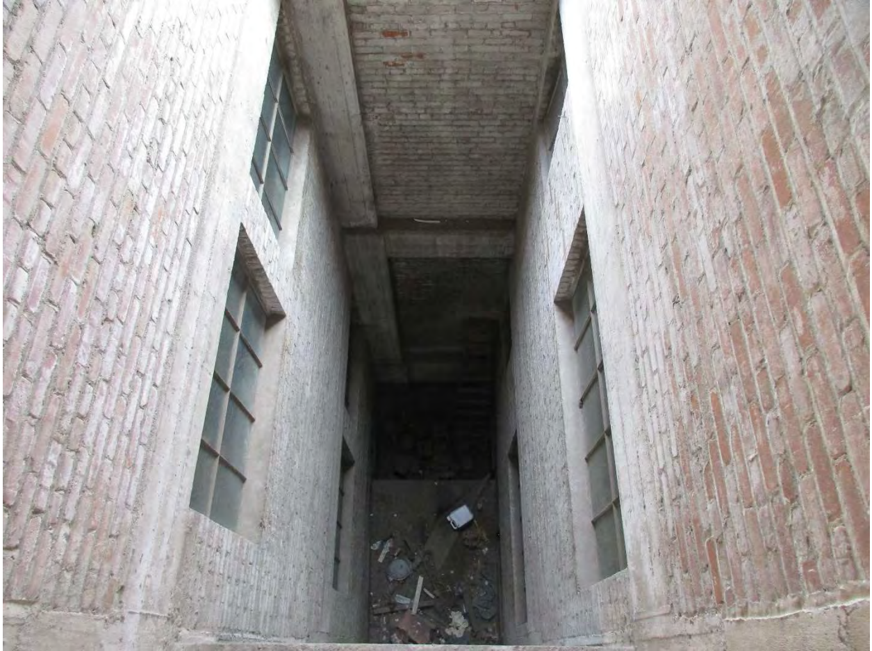
20 THE INTERIOR OF THE LIGHTWELL AT THE WEST SIDE OF THE EAST WING, LOOKING DOWN.
