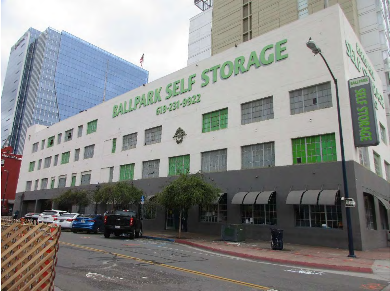
04 LOOKING SOUTH ACROSS ISLAND AVE. AT THE PRIMARY NORTH FAÇADE (w/o SCALE STICK).
