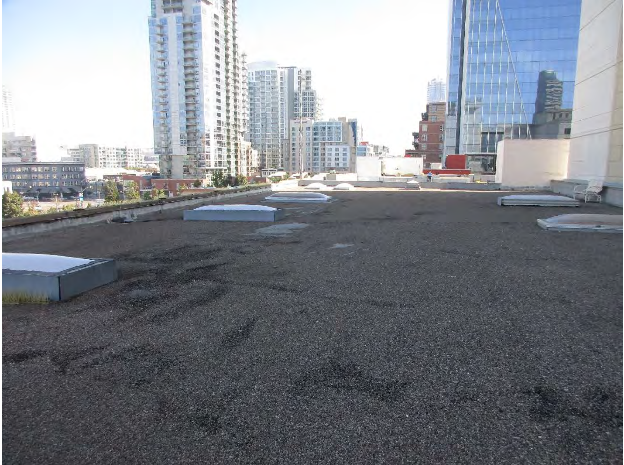
21 VIEW LOOKNG EAST OVER THE ROOF FROM THE WEST END OF THE WEST WING.
