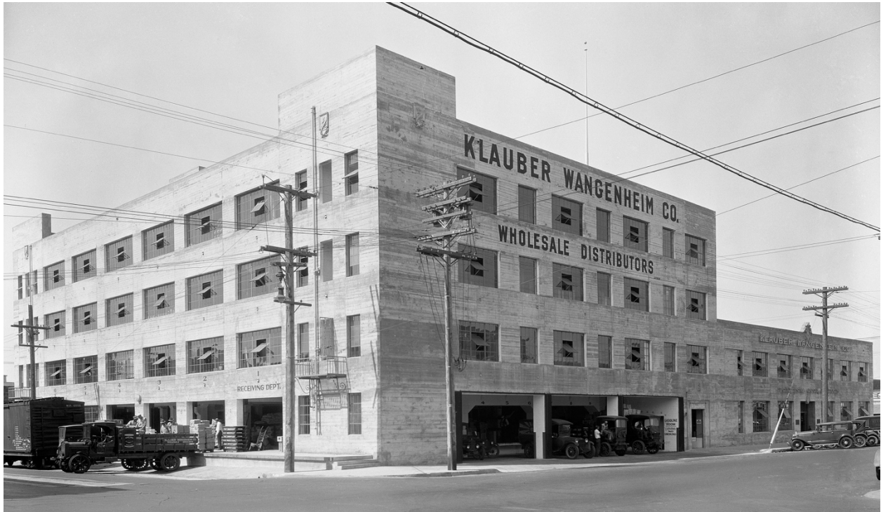
Figure 3: Historic photo of the Klauber-Wangenheim Building ca.1929 looking southwest. The original walls were unpainted tinted board-formed concrete. The painted signage on the building was likely black.
