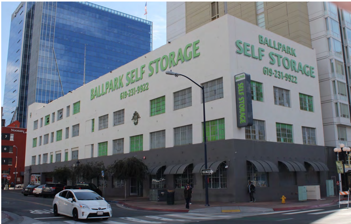
Figure 6: View of the Klauber-Wangenheim Building from 2020 looking southeast. Note the non-historic awnings.
