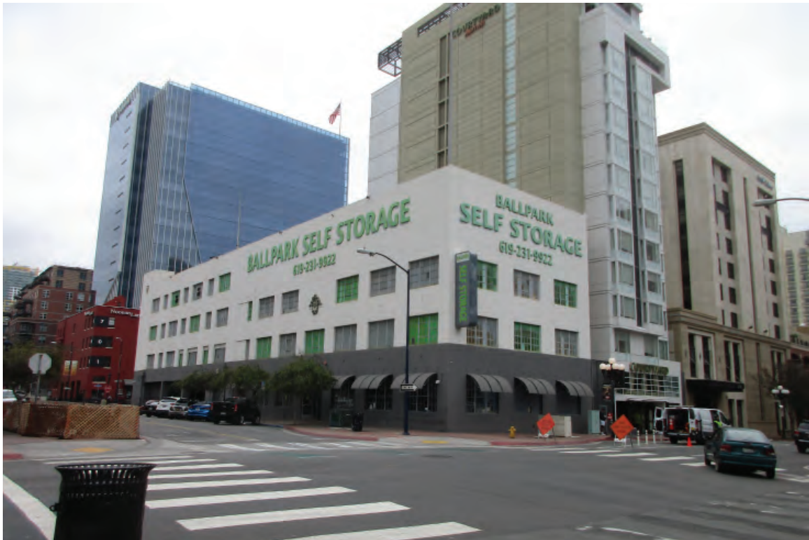
Figure 3-2: Looking southeast across the Island and Sixth Avenue intersection at the Klauber-Wangenheim Building.
