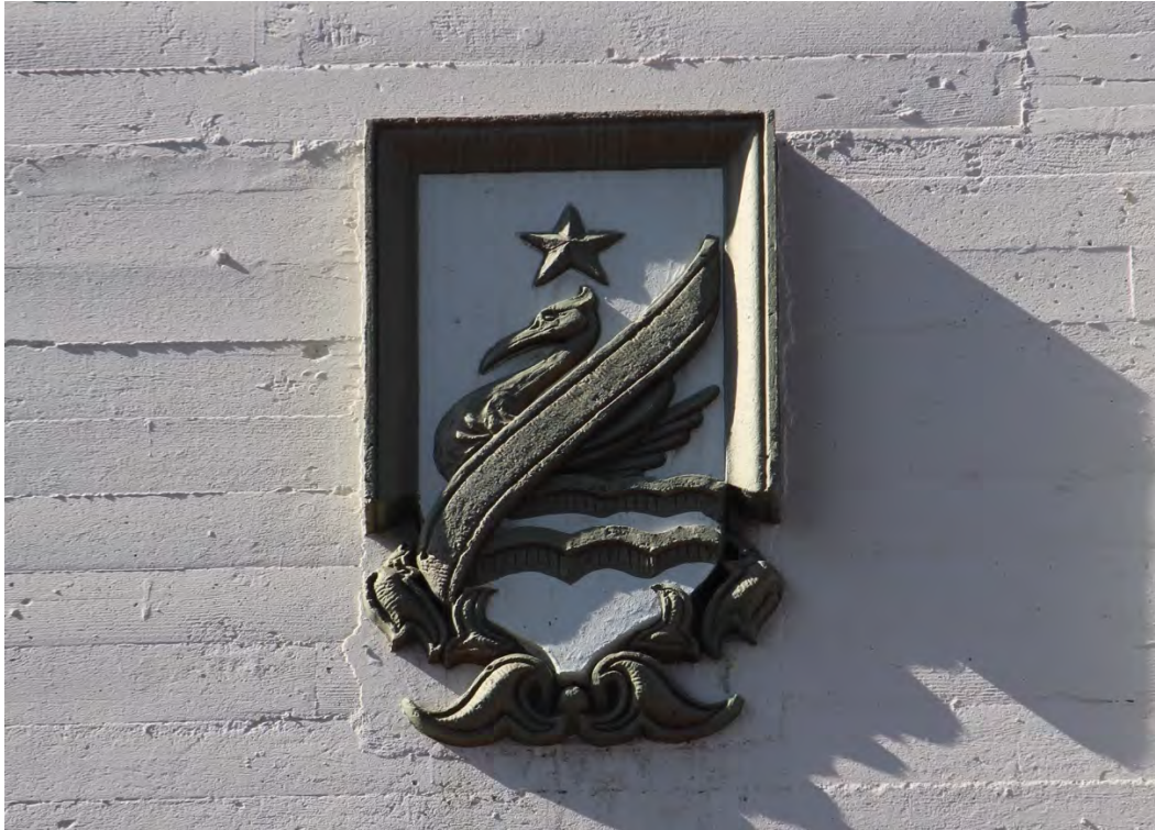
Figure 15: One of three cast-stone “pelican shields” that will be protected-in-place. Note the adjacent board-formed cast-in-place concrete wall finish.
