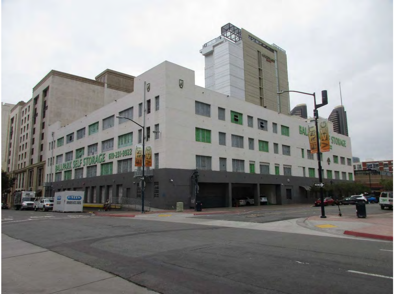
02 LOOKING SOUTHWEST ACROSS ISLAND AVE AND SEVENTH STREET INTERSECTION.
