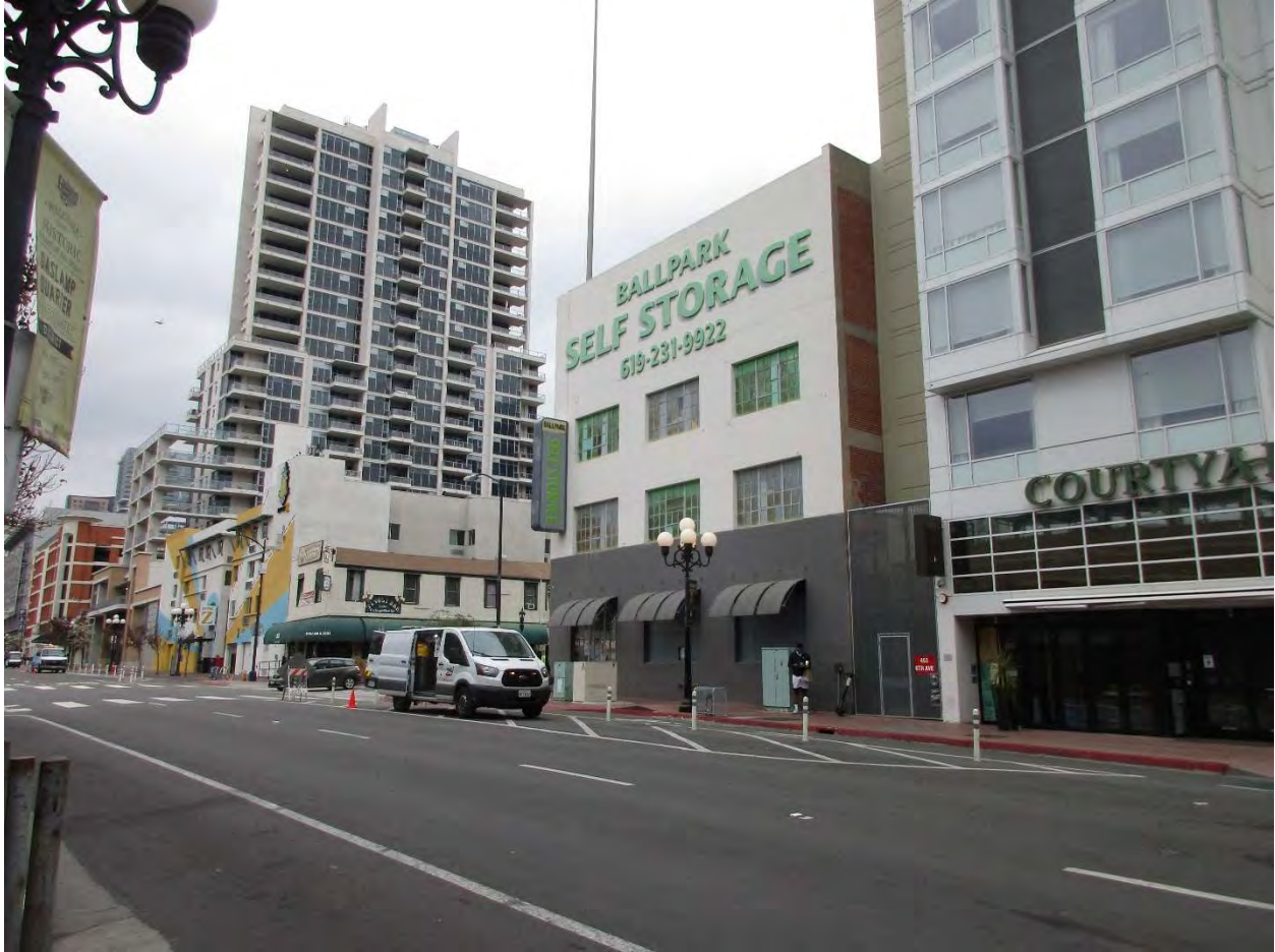
05 CONTEXT VIEW LOOKING NORTHEAST AT THE WEST FAÇADE. A SMALL PORTION OF THE SOUTH FAÇADE IS VISIBLE SHOWING THE CONCRETE POST AND BEAM FRAMING WITH BRICK INFILL.
