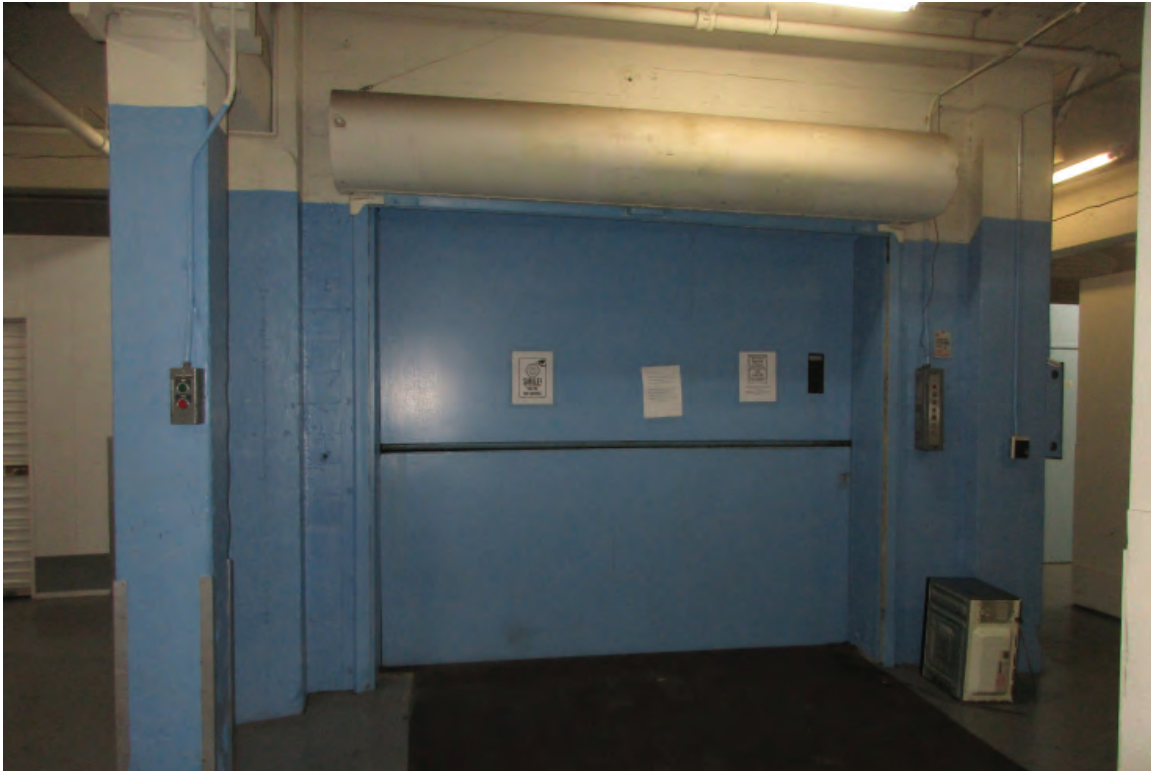
Figure 3-18: Second floor looking east at the east wing freight elevator.
