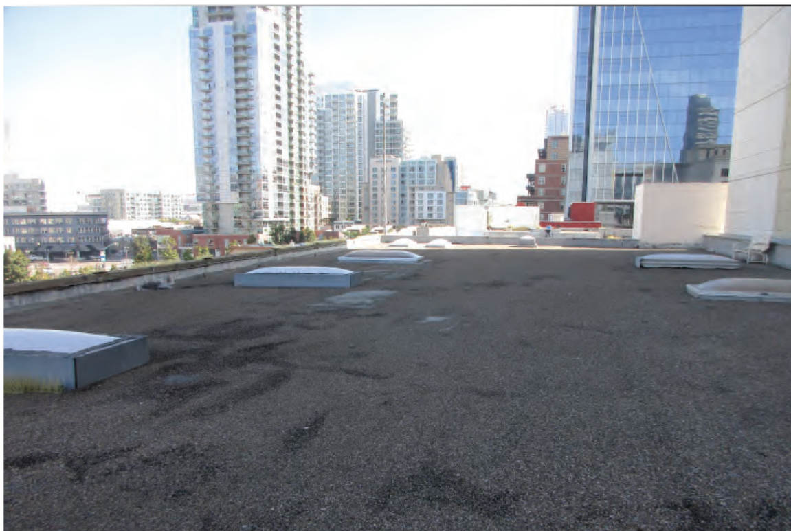
Figure 3-21: Looking east across the building's roof from the west wing.
