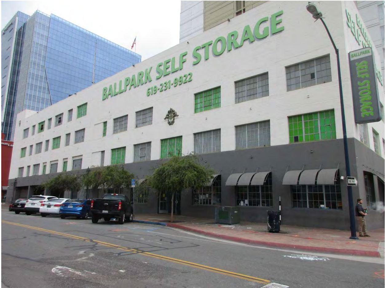
03 LOOKING SOUTH ACROSS ISLAND AVE. AT THE PRIMARY NORTH FAÇADE (WITH SCALE STICK).
