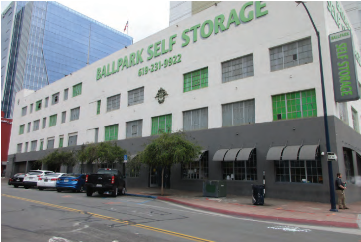
Figure 3-4: Looking south across Island Avenue at the primary north façade.
