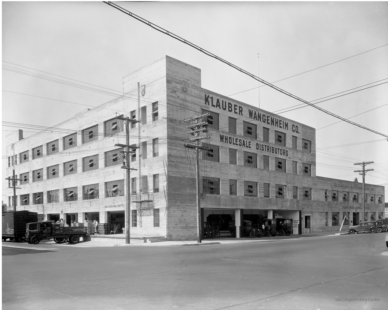
H1 LOOKING SOUTHWEST ACROSS ISLAND AVE. AT THE NORTH AND EAST FAÇADES OF THE KLAUBER WANGENHEIM CO., DATED CA.1929. NOTE THE TWO-STORY WEST WING PRIOR TO THE TWO-STORY ADDITION. SOURCE: SAN DIEGO HISTORY CENTER.
