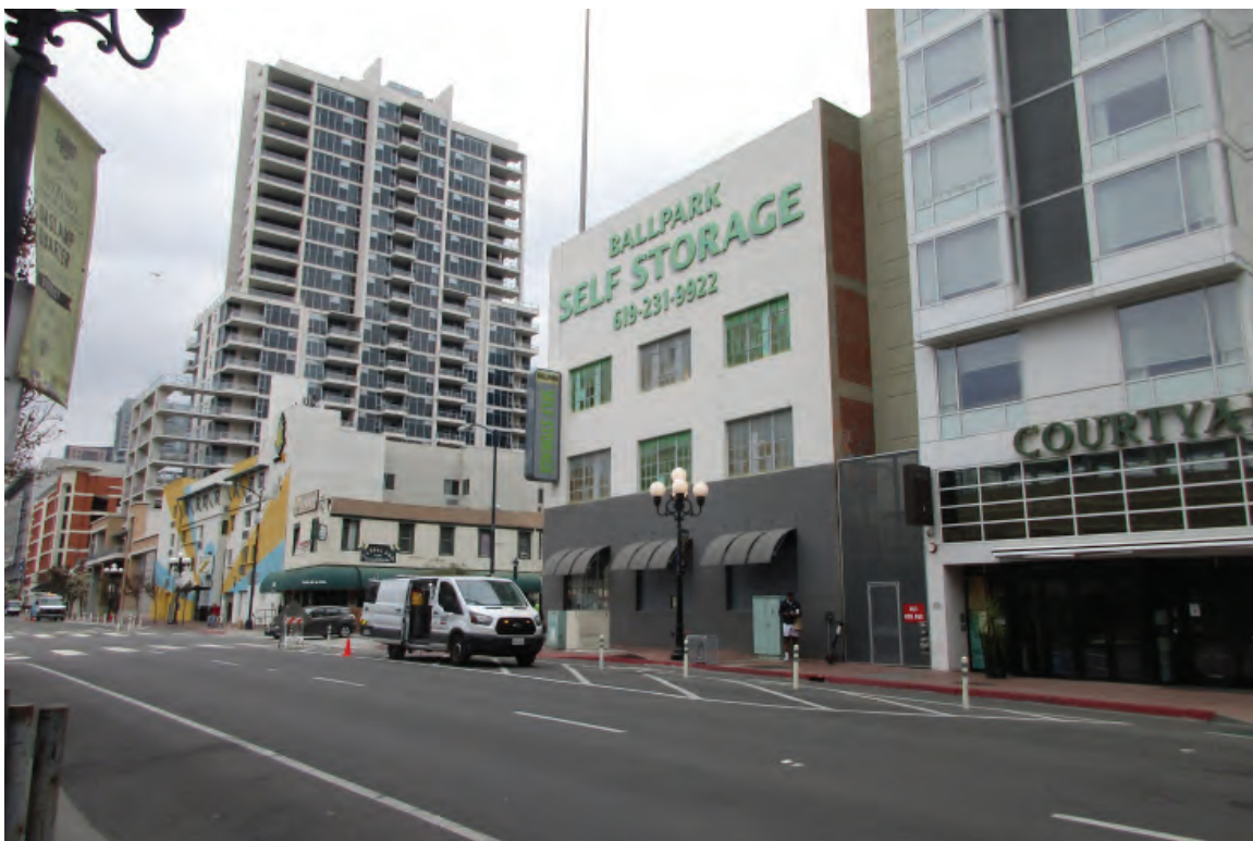
Figure 3-5: Context view looking northeast at the west façade. A small portion of the south façade is visible showing the concrete post and beam framing with masonry infill.
