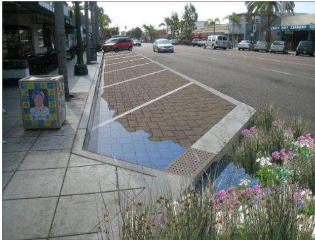
Figure I-5. Permeable pavement parking area in the right-of-way
