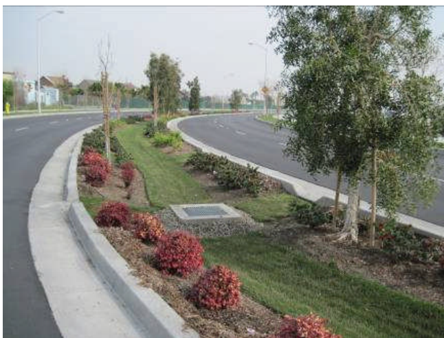
Figure I-3. Road median bioswale
