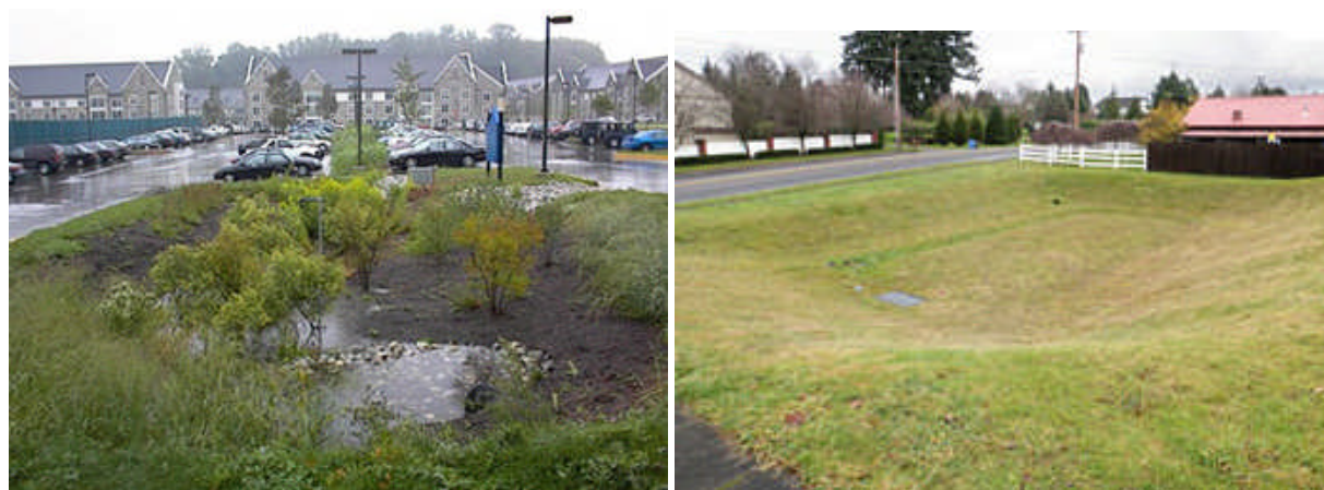
Figure I-12. Typical surface infiltration basins
