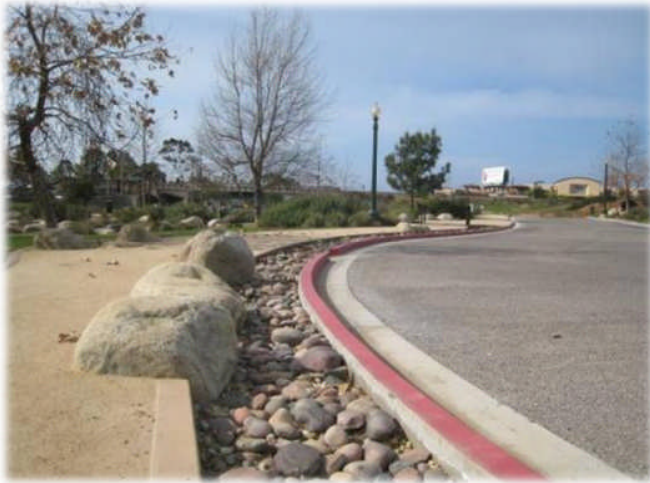
Figure I-2. Infiltration trench
