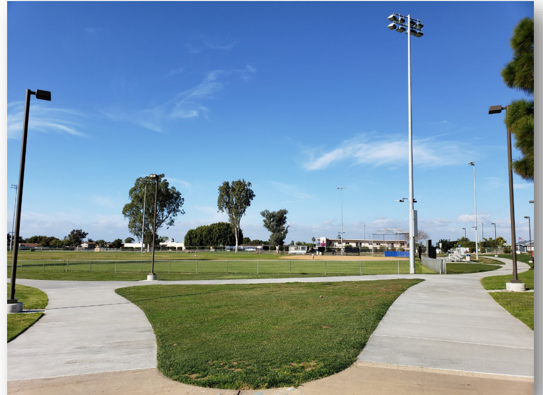
Silver Wing Park Ballfield Lighting Phase II
