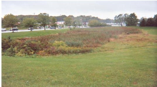
Figure 1. Example of a Dry Extended Detention Basin
