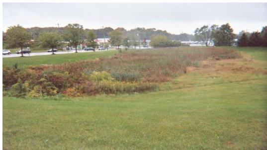
Figure 1. Example of a Dry Extended Detention Basin
