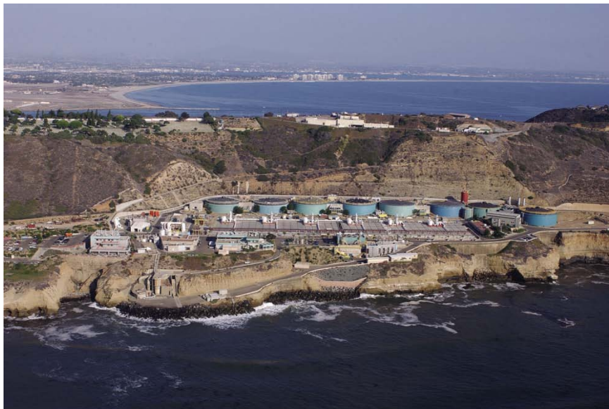
The Point Loma Wastewater Treatment Plant is the terminal treatment facility serving a Metro System population of approximately 2.2 million.
