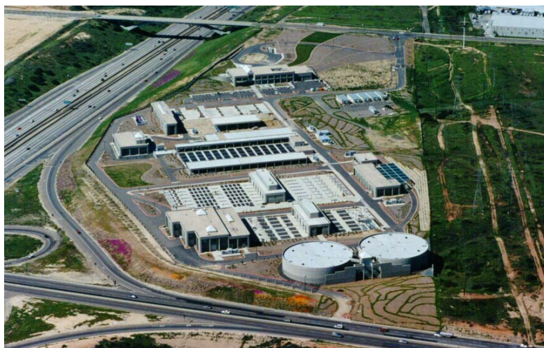
The North City Water Reclamation Plant produces a high quality recycled water supply that complies with State of California standards for all irrigation uses.
