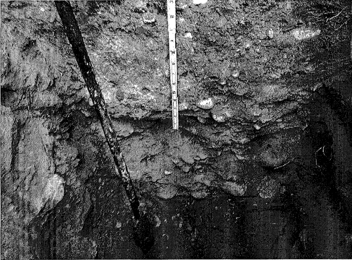
PHOTO 1: Bottom of Footing at Test Pit P-1.
