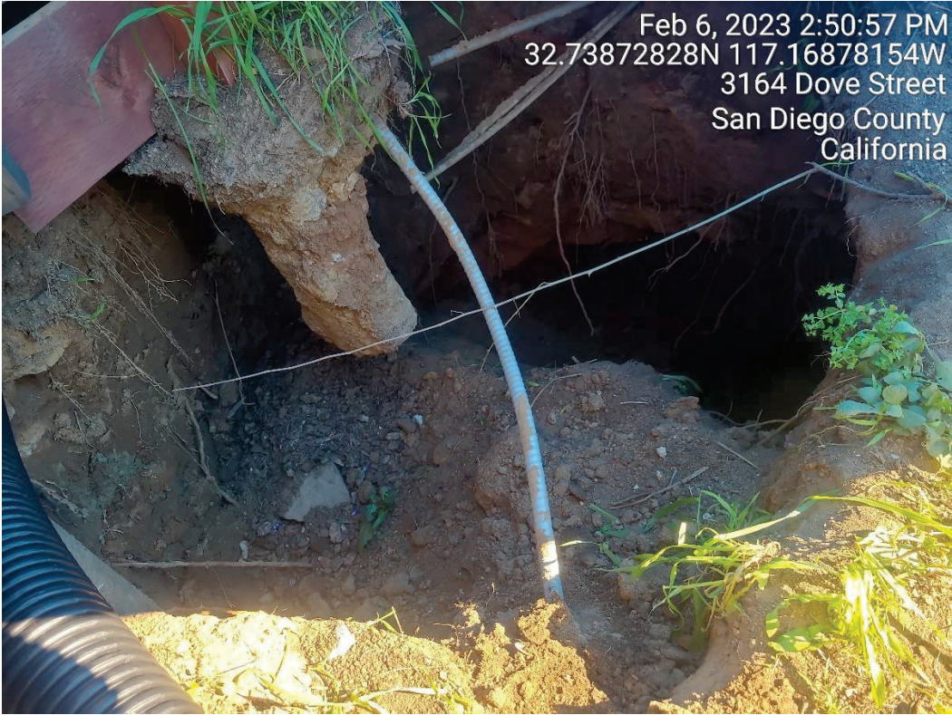
Figure 2 - Exposed Foundation
