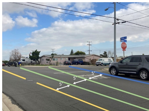
Non-conforming utility separation along Triton Avenue with two sewer mains.
