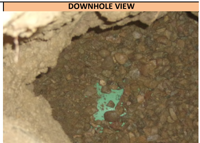
A downhole view of the SDR-35 sanitary sewer utility found in Pothole 9 at the depth of 81 inches T/P. Utility runs in a NE/SW direction at the pothole location and was found directly on markout.
