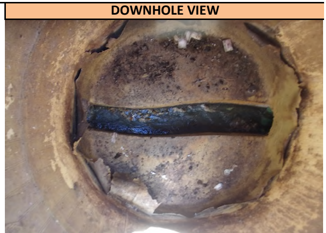
A downhole view of the utilities found in Manhole1 and their orientation at the pothole location: an 8 inch PVC sanitary sewer utility at the depth of 76 inches T/P; and a 6 inch PVC sanitary sewer utility at the depth of 74 inches T/P. Flow line is east to west.
