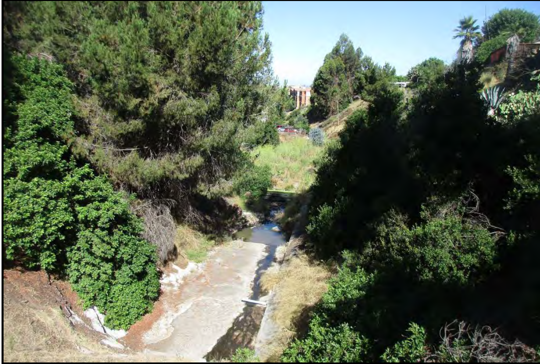
PHOTOGRAPH 3 Slope West of 54th Street, Looking West
