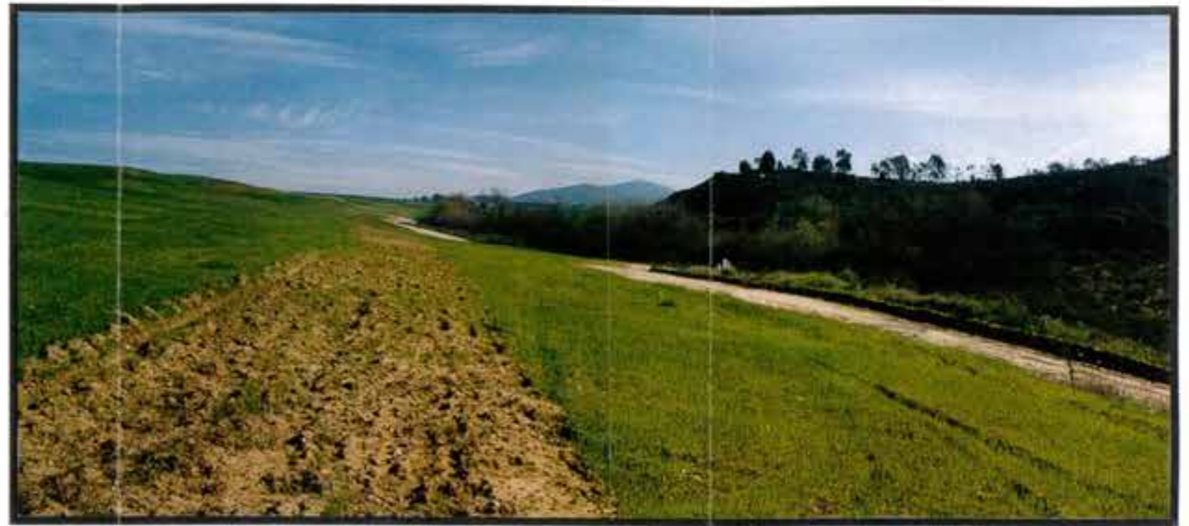
PHOTOGRAPH 4E-16 Looking East along Gonzales Canyon/Urban Amenity
