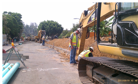
TCDB installs deep sewer mains in a residential neighborhood.
