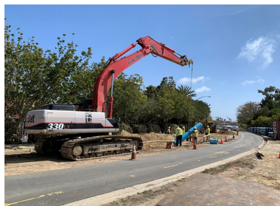
16” PVC Installation along La Jolla Scenic Drive.
