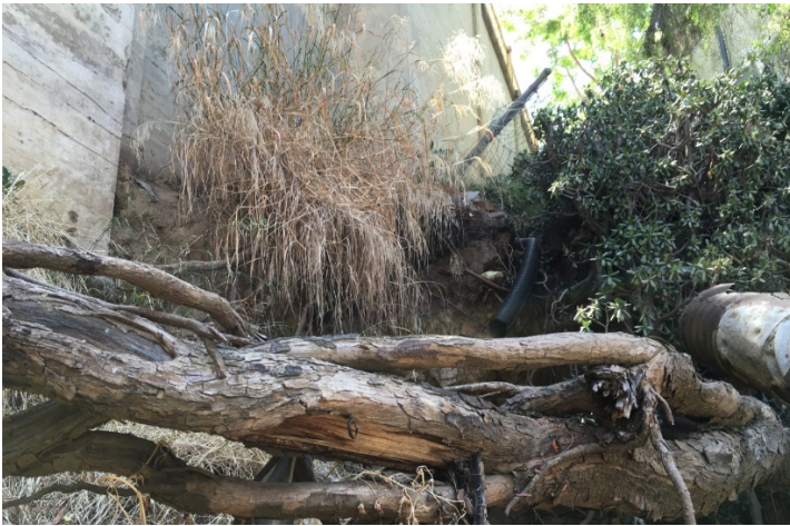
TAKEN FROM THE SINKHOLE LOOKING SOUTHEAST
