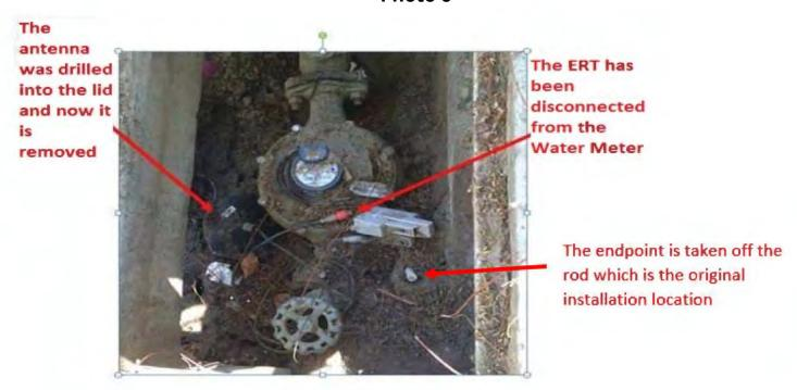
Sewer Group Job 843 Appendix L - Advanced Metering Infrastructure (AMI) Device Protection You are responsible when working in and around meter boxes. If you encounter these endpoints, use proper care and do not disconnect them from the registers on top of the water meter. If the lid has an antenna drilled through, do not change or tamper with the lid and inform the Resident Engineer immediately about the location of that lid. Refer to Photo 7 below:
