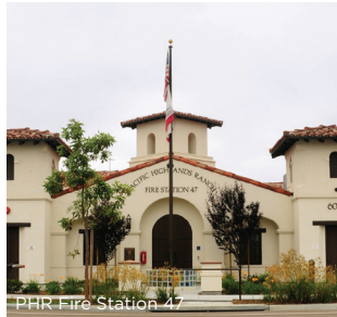
PHR Fire Station 47
