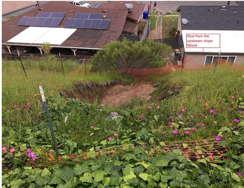
Existing Slope Failure
