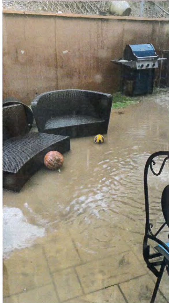
Photo 10 – water ponding in the backyard.
