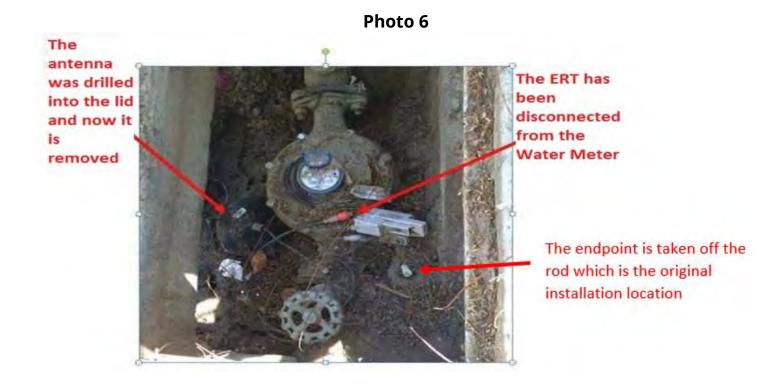
You are responsible when working in and around meter boxes. If you encounter these endpoints, use proper care and do not disconnect them from the registers on top of the water meter. If the lid has an antenna drilled through, do not change or tamper with the lid and inform the Resident Engineer immediately about the location of that lid. Refer to Photo 7 below:
