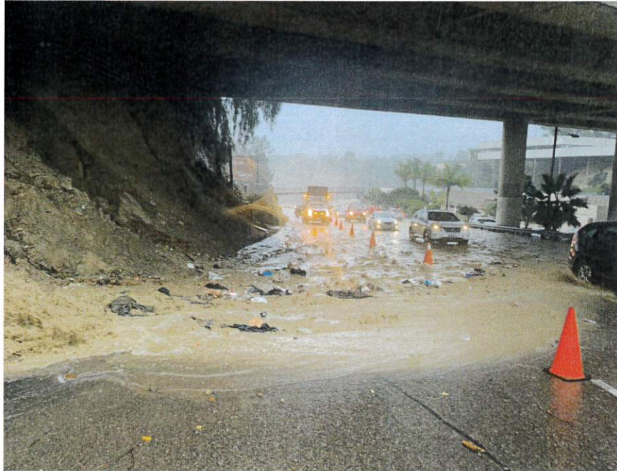
6 th Avenue underneath Washington Street Bridge
