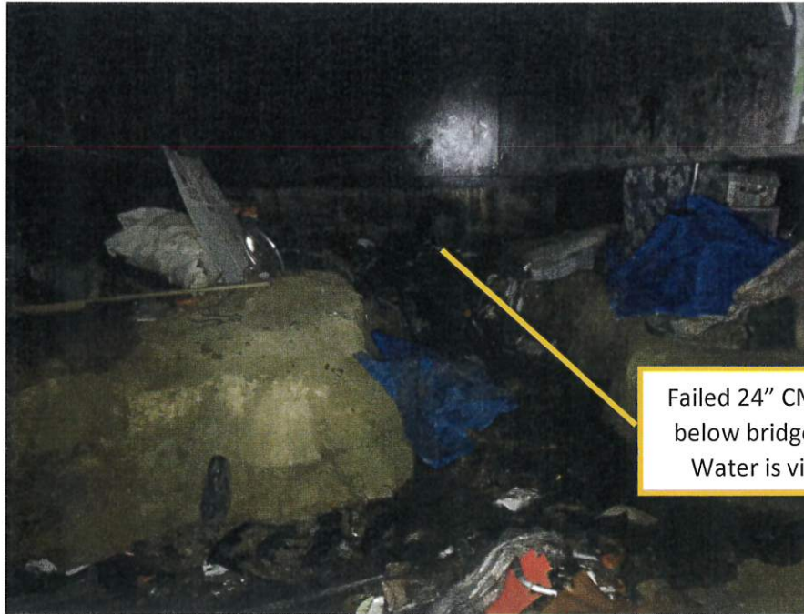
View just below Washington Street Bridge deck
