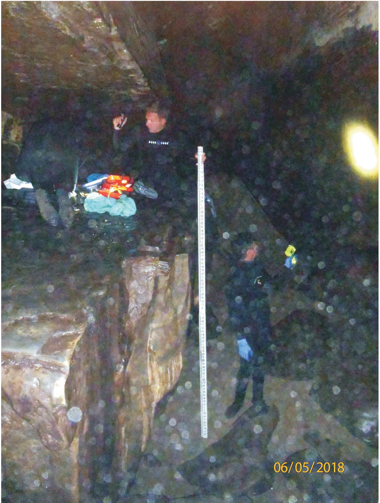
PHOTO 3: MAIN BLOCK SEEN IN 2002 SURVEY STILL MOSTLY INTACT. A CAVITY HAS DEVELOPED, UNDERMINING THE SOUTHERLY SIDE OF THE BLOCK.
