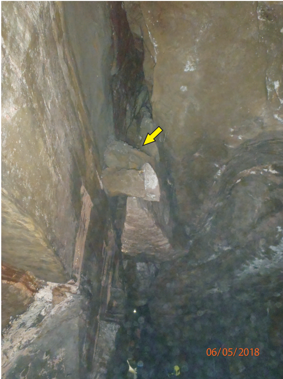
PHOTO 6: ARROW INDICATES DOWN DROPPED BLOCK. NOTE SAND ON TOP OF BLOCK.
