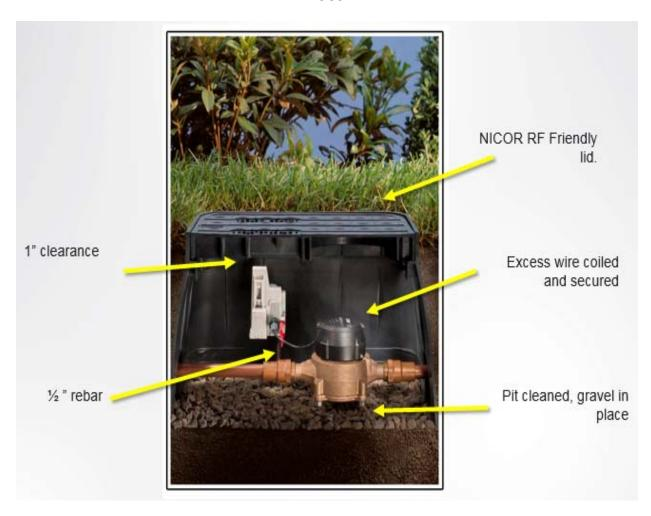
The AMI device ERT/Endpoint/Transmitter shall be positioned and installed as discussed in this Appendix. If the ERT/Endpoint/Transmitter is disturbed, it shall be re-installed and returned to its original installation with the end points pointed upwards as shown below in Photo 5.
