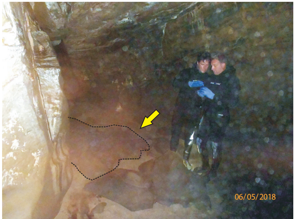
PHOTO 5A: NOTE APPARENT RECENT ROCK DEBRIS (ARROW).
