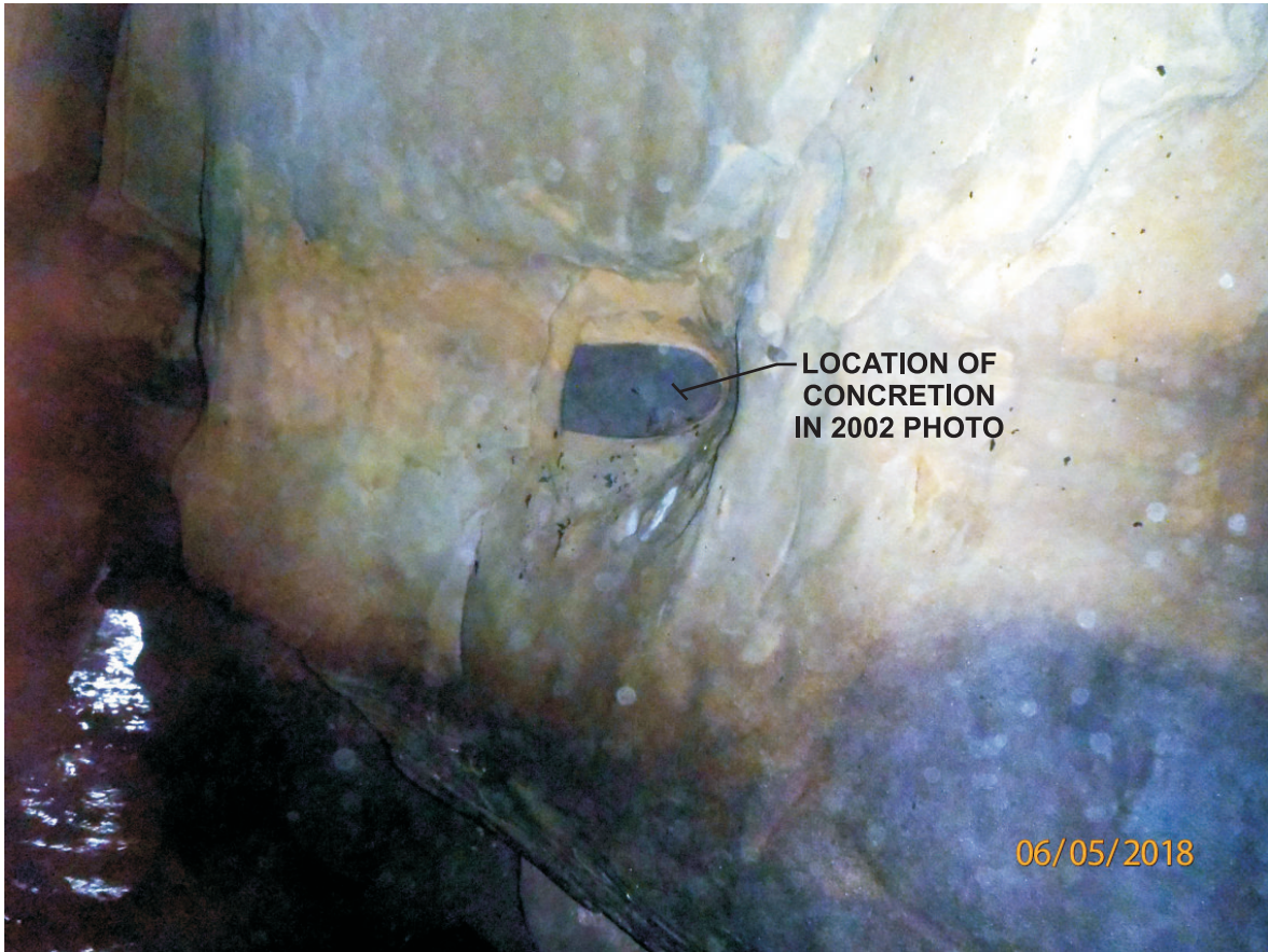
PHOTO 2: NOTE LARGE CONCRETION IS GONE, AND WALLS HAVE ERODED BACK AND WIDENED.
