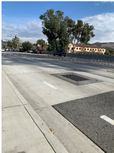
Figure 5: Example of vaults for Flex Tend joints
