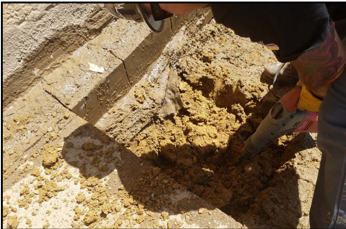
Figure 3-2. Footing Inspection Trench
