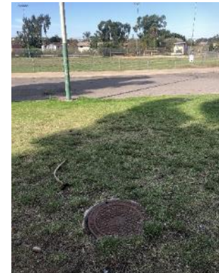
Figure 5 Manhole upstream of segment L61
