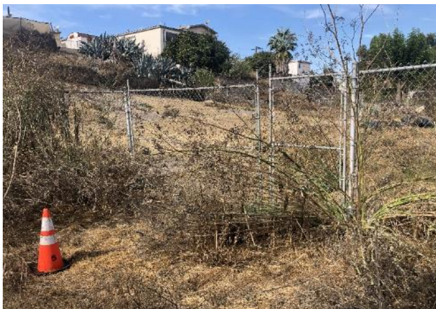
Figure 8 Lot containing one of the manholes to be accessed for rehabilitation work
