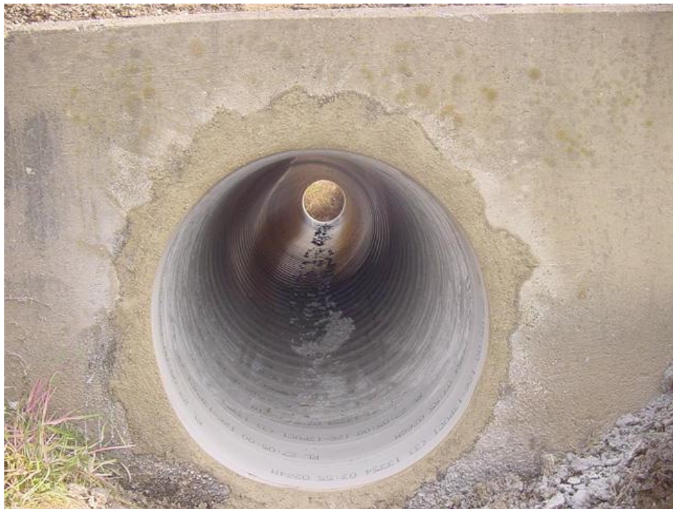
Figure 7: Culvert after rehabilitation
