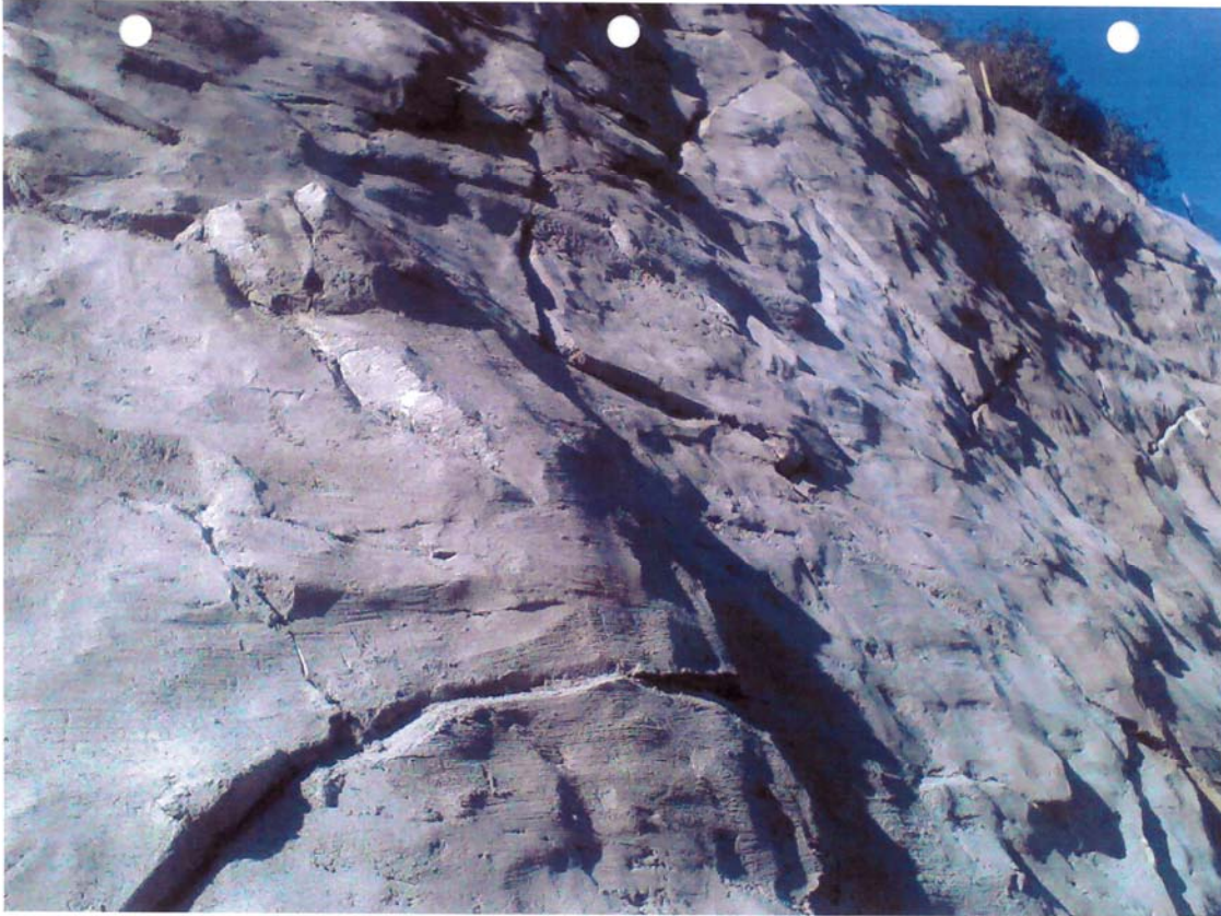
SOIL NAIL WALL - TEXTURE
