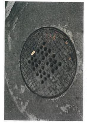
Figure 6: SDG&E manhole cover for underground transformers, Ridgeway, July 2010
