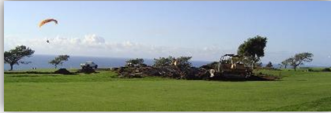
LU Torrey Pines South Course renovation 2005-2008 prior to 2008 US Open
