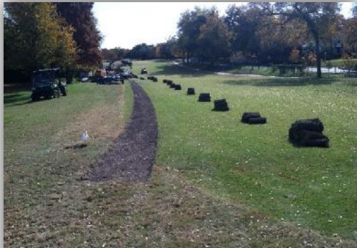
Sod cut, rolled and moved away for mainline trenching
