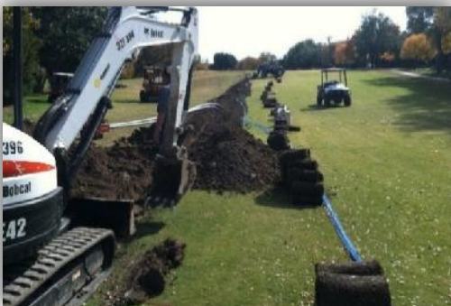
Rubber track mini-ex utilized for mainline trenching
