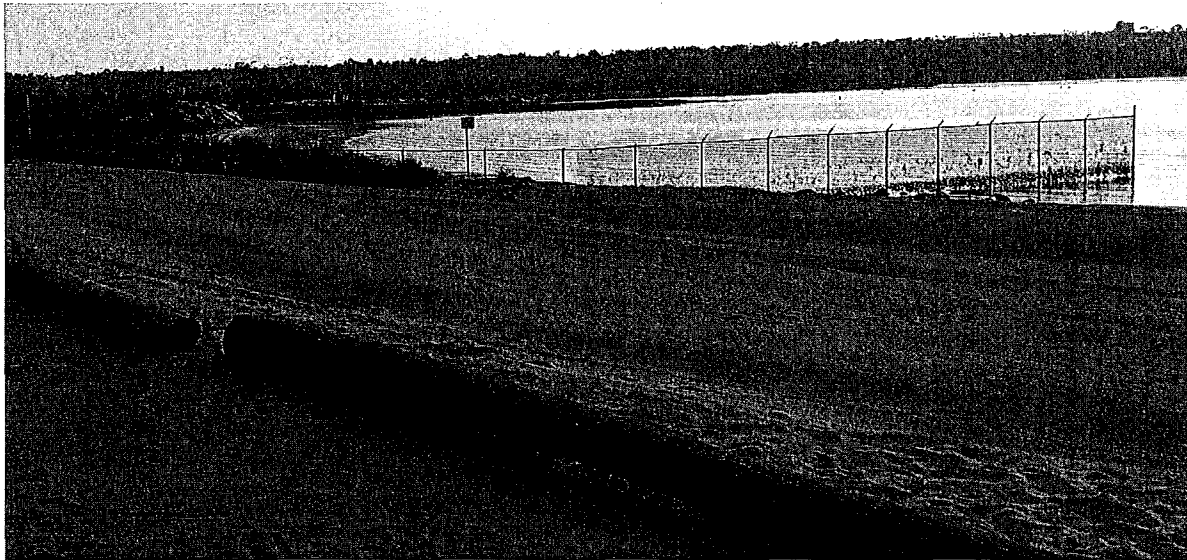
Photograph 11. View to the northeast at the north end of Crown Point Shores adjacent to the Stribley Memorial Marsh. Sand at this site has accumulated around and over the existing access barrier fence resulting in lowering the effective fence height to as little as 3 feet in some areas. (08-09-16)
