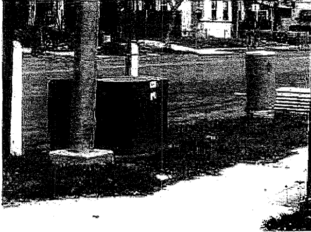
Figure 1.2: Vandalized transformer box, Talmadge, May 2010
