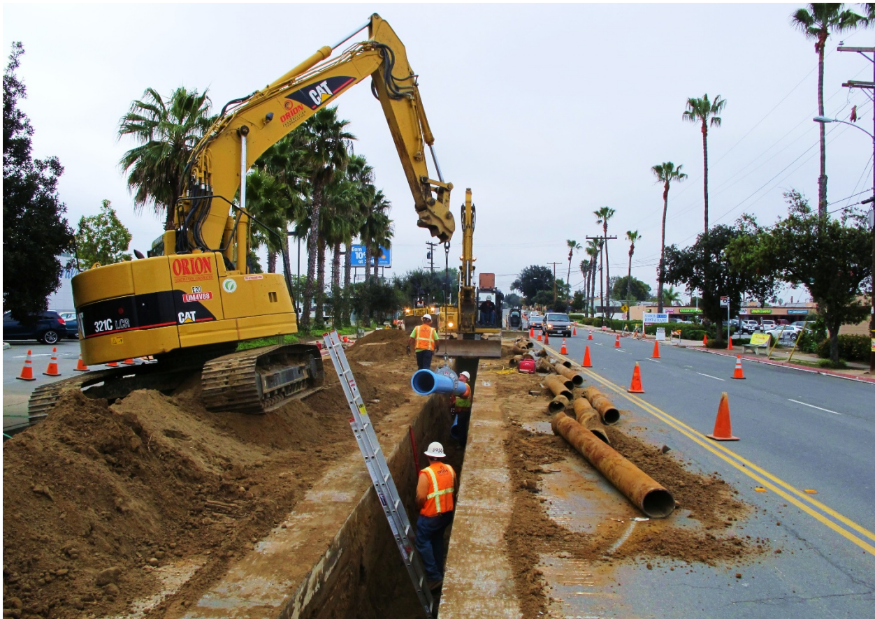
Orion waterline installation crew installs new, PVC waterline in San Diego.
