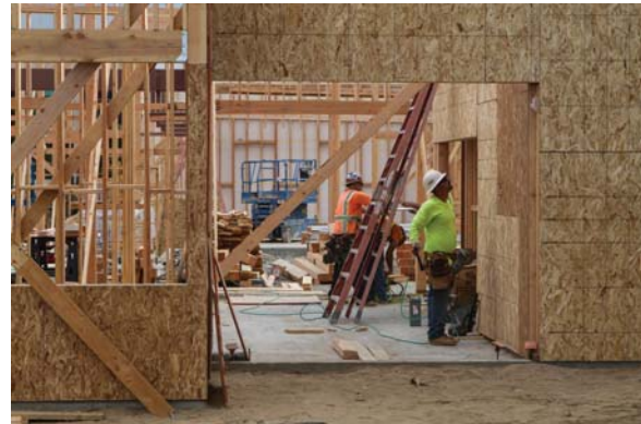
City of Coronado John D. Spreckels Center Under Construction, August 2016
