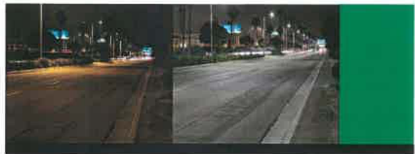
Figure 4: Port of San Diego LED Lighting Retrofit
