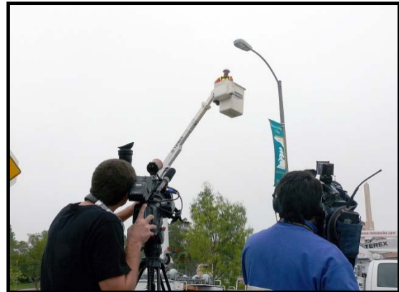
First light installed in San Diego
