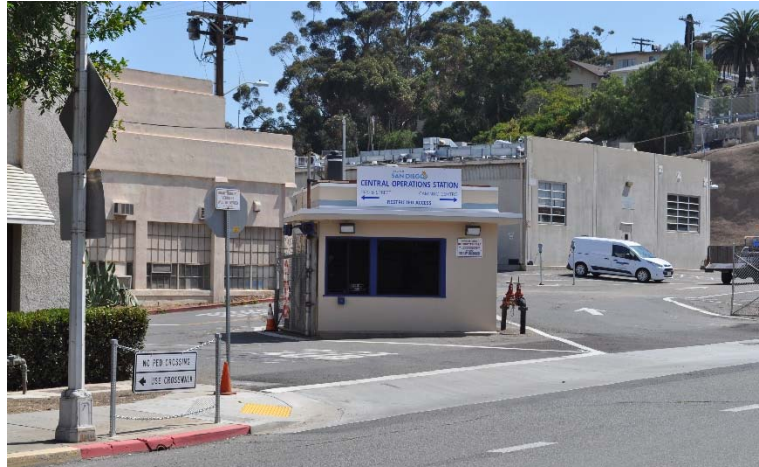
City Operations Station at B Street
