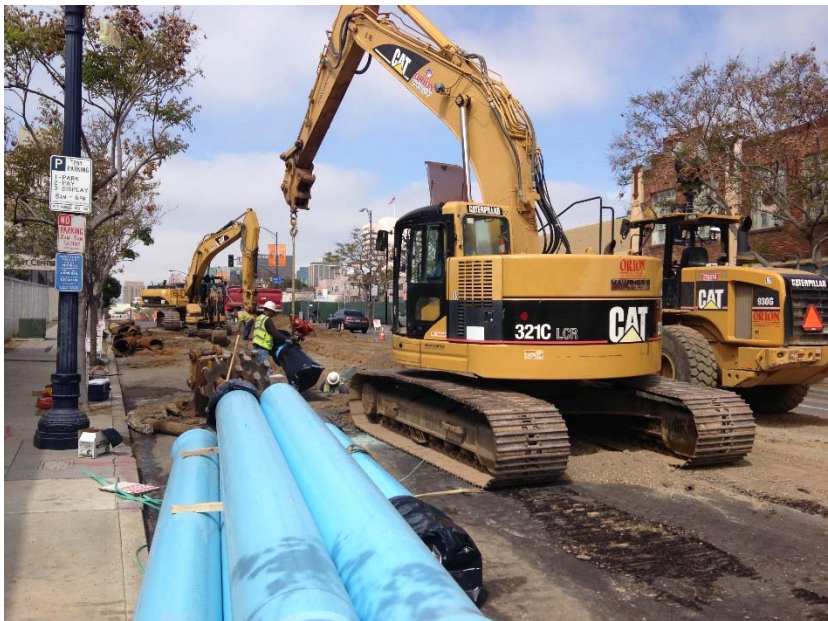
16" Replace in Place Pipe
