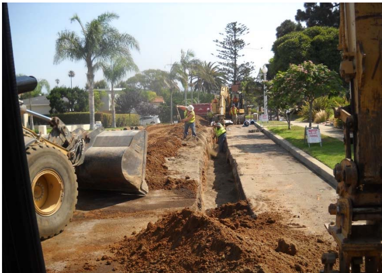
Replace in Place Pipeline Install
