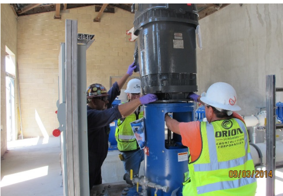
Setting Pump Motors
