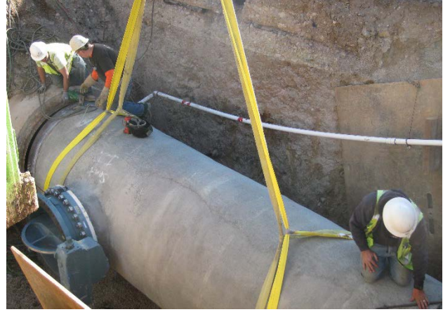
Laying Yard Piping
