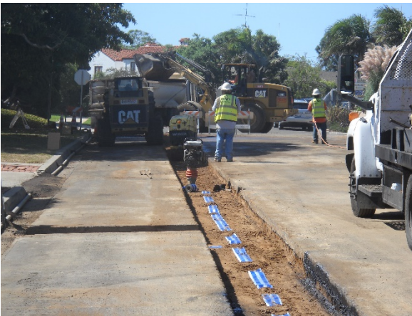
Trench Backfill
