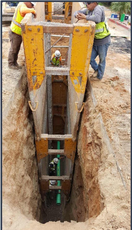
20' Deep sewer installation
