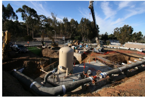
Surge Tank Installation
