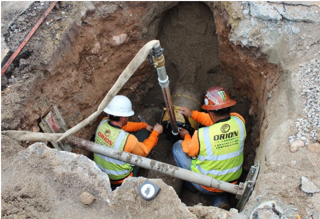
Flushing and Testing
