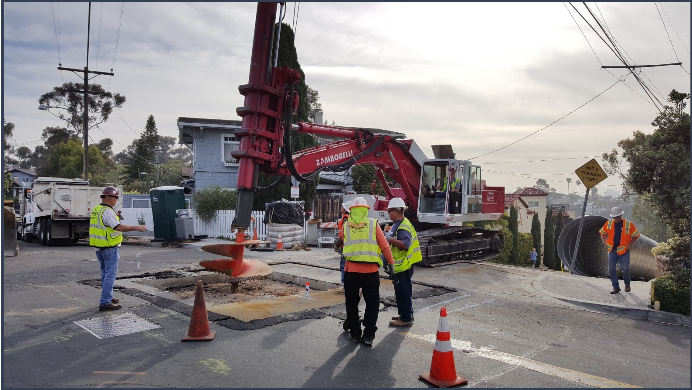
Crews installing CMP shafting at the Pringle Street location
