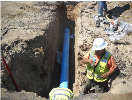
PVC Pipe Install
