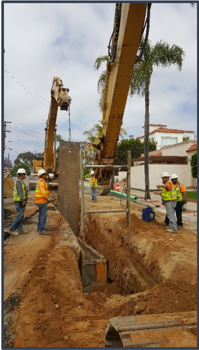
Stacking Trench Shields
