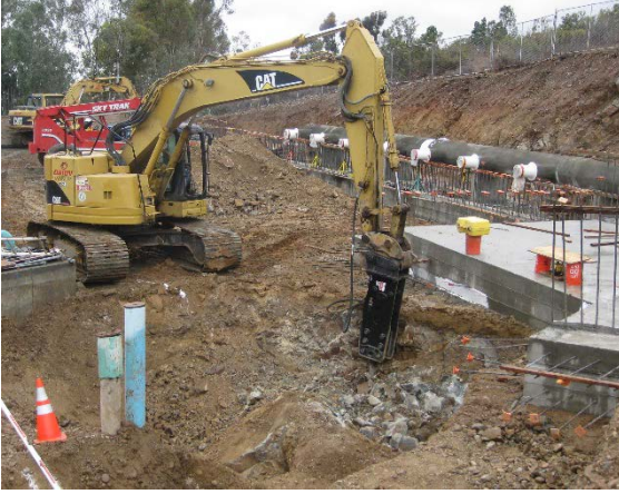
Excavating Pipe Trench
