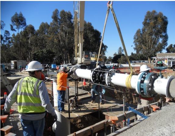
Installing Discharge Piping
