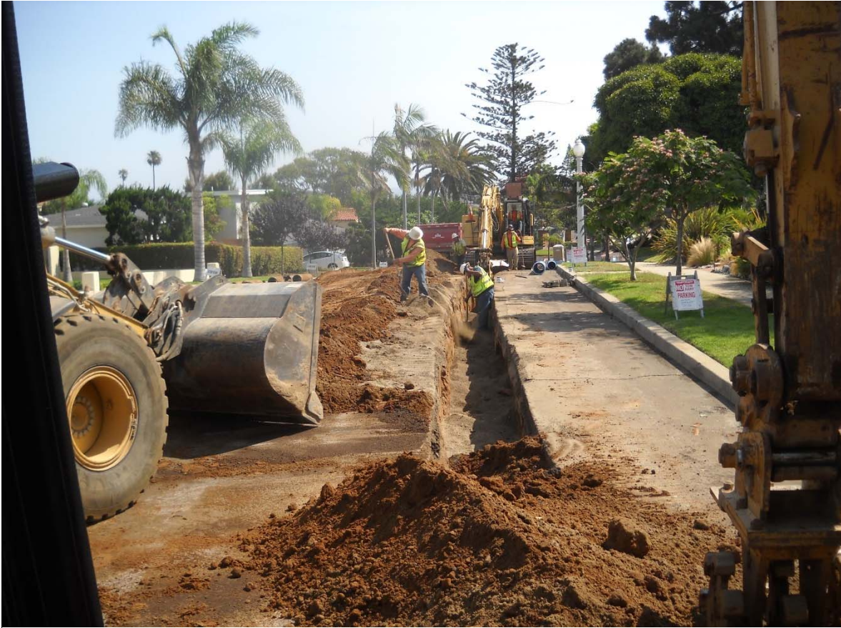
Back fill with sand around the new PVC pipe.
