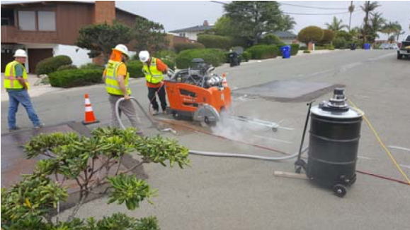
Orion Crews sawcutting trench.
