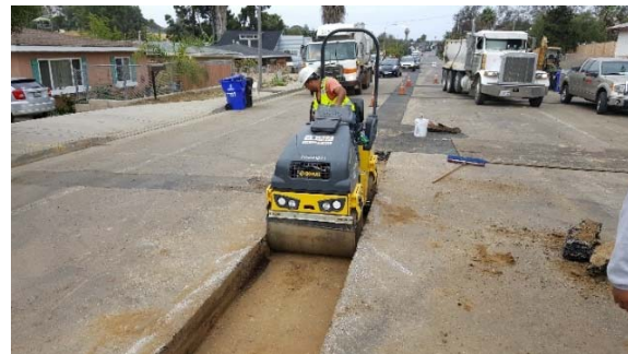
Orion crews base paving trench
