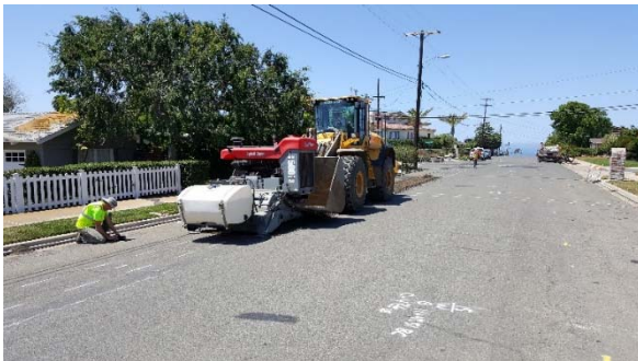
Orion crews grinding asphalt with company owned equipment
