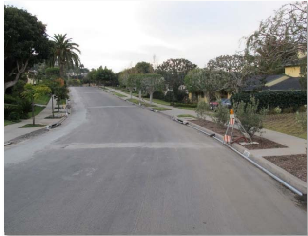
Figure 8 – High-lining on a Residential Street
