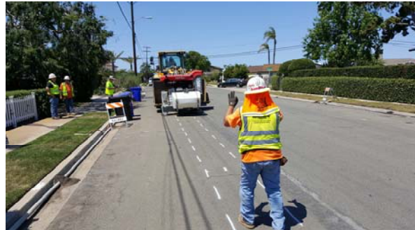
Orion crews grinding asphalt
