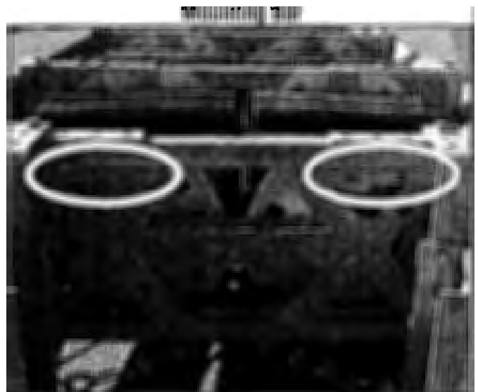
EAEs Secured with Mounting Bars
