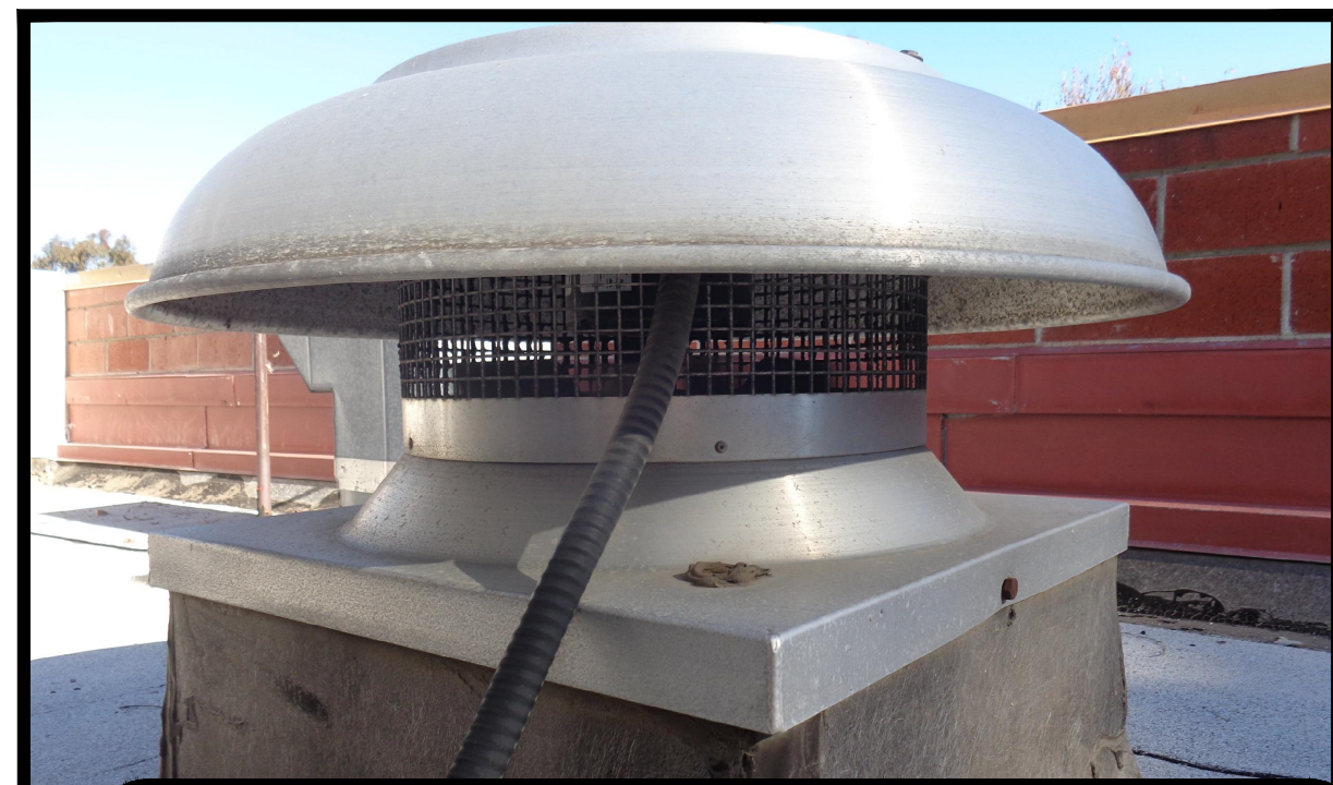
6 TYPICAL ROOF MOUNTED EXHAUST FAN TO BE REPLACED.
