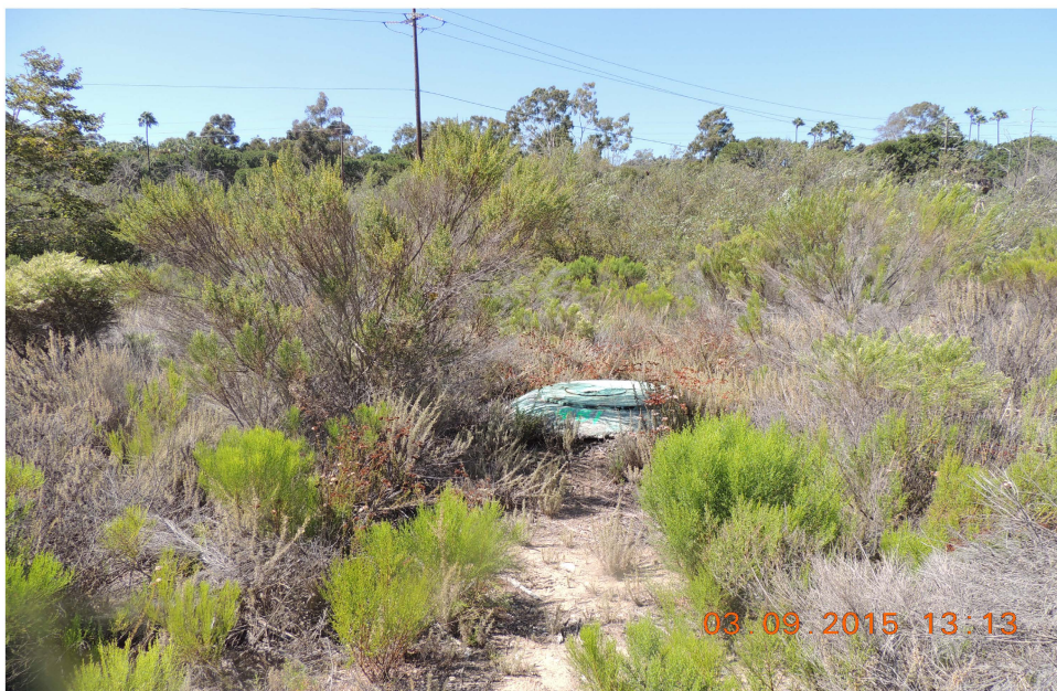
Manhole number 464 in coastal sage scrub dominated by broom baccharis.
