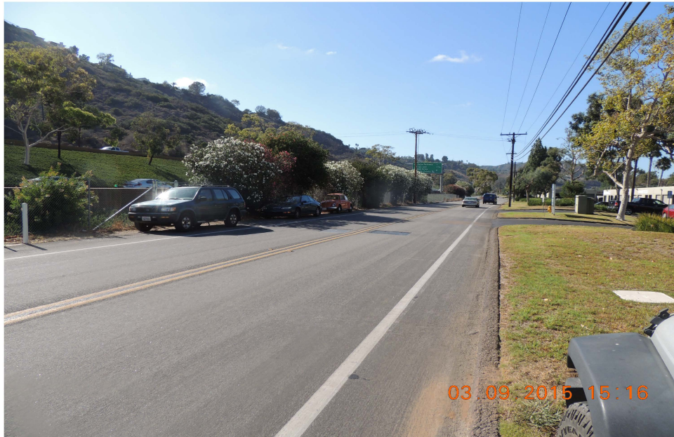
Manhole number 377 is in a developed road with no state or federal jurisdictional waters.
