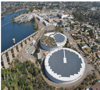
Alvarado Water Treatment Plant San Diego, CA
