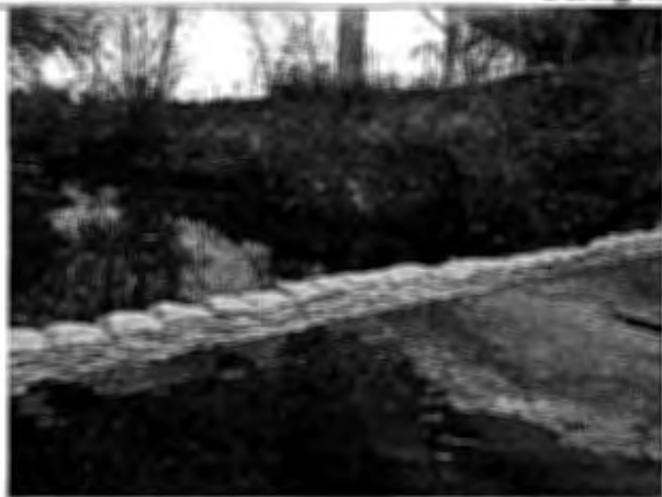
Jan 29, 2016. Upstream sandbag berm set up
