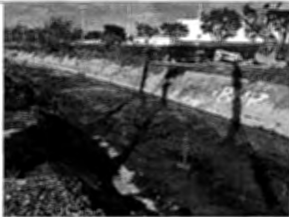
Feb 1, 2016. Middle portion of emergency work area, facing downstream
