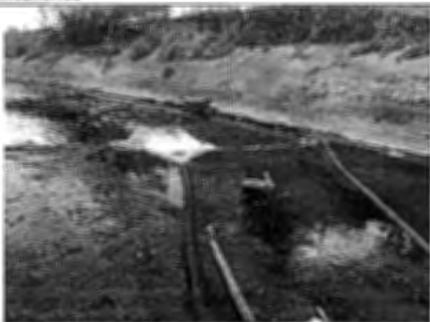
Jan 29, 2016. Diversion hose set up
