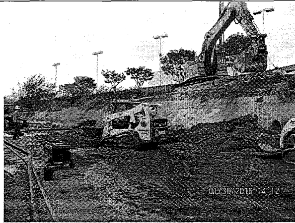
Jan 30, 2016. Middle portion of emergency work area, facing downstream
