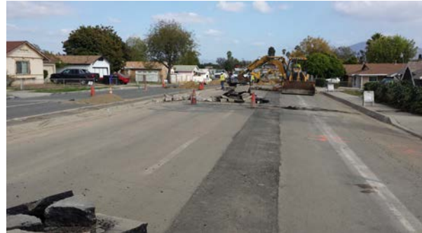
TCDB Team water service and appurtenance crews working on laterals for completed mainline.
