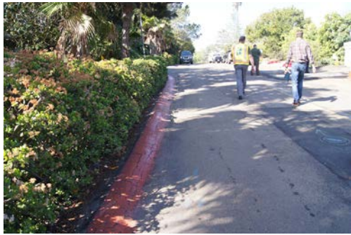
Many streets along the project alignment do not have sidewalks.
