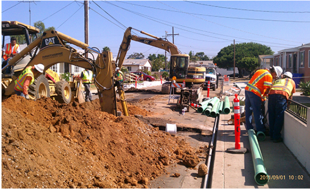
Installation of deep sewer mains, with water highlined in advance. Onsite TCDB huddle with City staff handling unknown utility conflicts while work is in progress.
