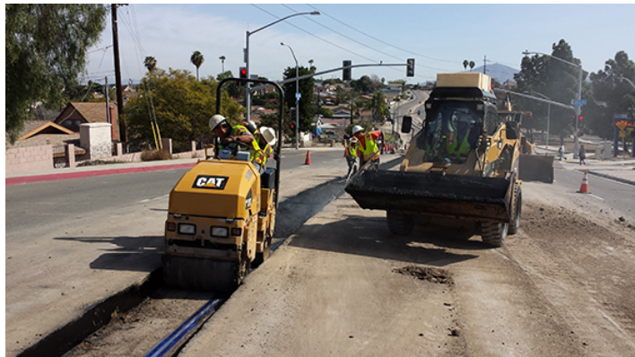
Deep lift permanent trench patching per SDG 107 Type 1 - MACC 1, Task Order 1.
