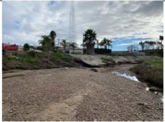
Photo Point 1 – Post-maintenance: Looking south within National 1 from below the National Ave. bridge at post-maintenance conditions (January 17, 2022)
