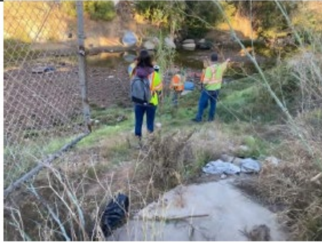
Photo Point 3 – Pre-maintenance: Looking northwest at access ramp prior to the start of maintenance (October 21, 2021).
