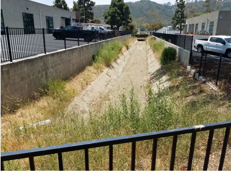
Flintkote pre-maintenance photo at the eastern terminus looking towards Roselle Street, illustrating primarily silt and vegetation growth along the upper bank (June 25, 2022)
