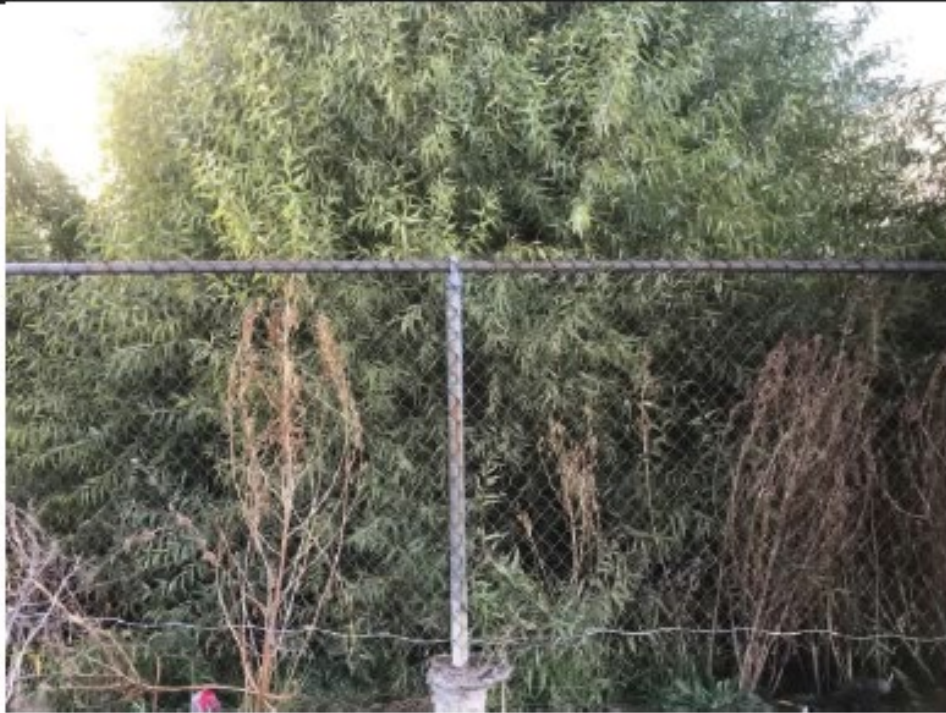
Pre-Maintenance Photo Point 4: Looking north from the southern end of Camino del Arroyo 1 – thick willow scrub/trees and vegetation shown within the channel (12/09/2021).
