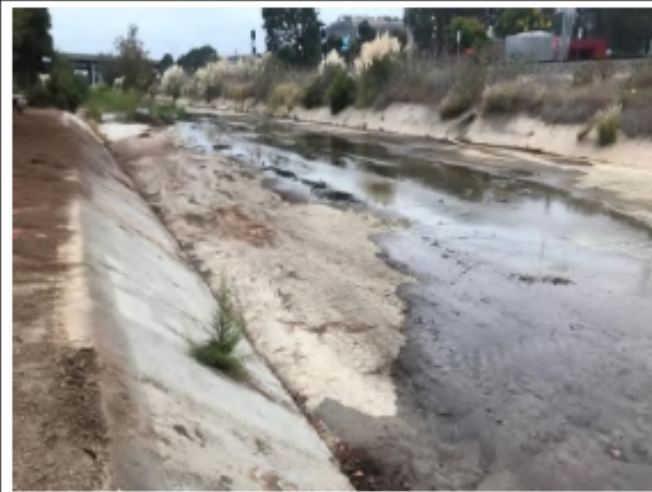
Roselle Pre-Maintenance - Photo 12: view of Roselle 2 looking north from southern end of maintenance area. Sediment and vegetation shown in channel bed.
