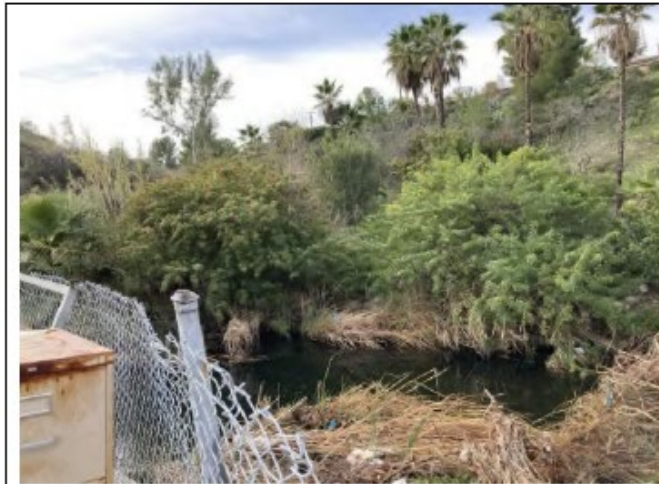
Photo Point 3 – Pre-Maintenance: Looking southwest within Alvarado 1 from the staging area at overgrown vegetation along the banks of the channel (January 26, 2022).
