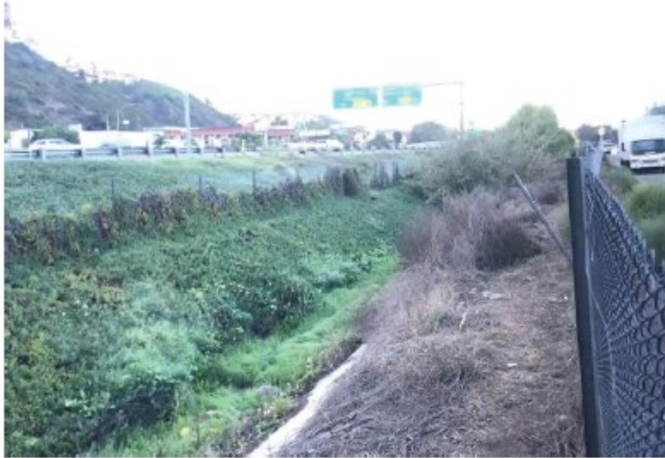
Pre-Maintenance Photo Point 6: Looking southwest from north bank of Camino del Rio 1 at vegetation and other materials accumulated in the downstream section of the channel (12/11/2021).
