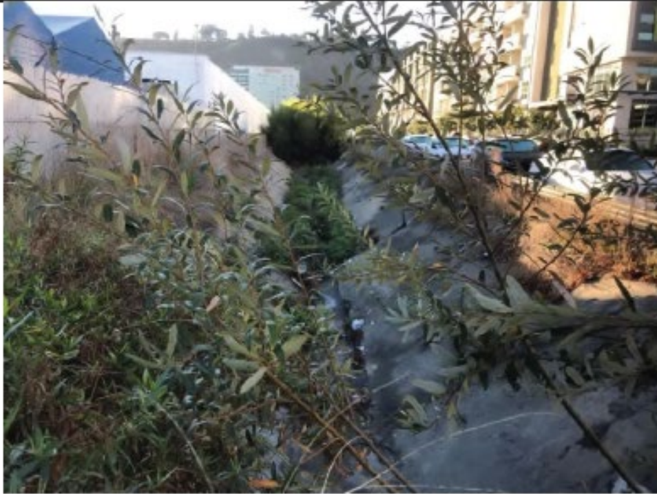
Pre-Maintenance Photo Point 1: Looking south from the northern, downstream end of Camino del Arroyo-vegetation and willow scrub/trees visible within the channel (12/11/21).
