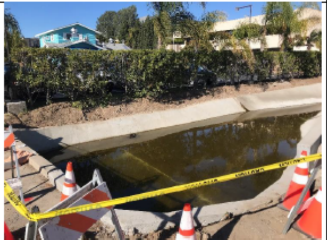
Post-Maintenance - Photo Point 4: Post-maintenance photo facing northeast from Sorrento Valley Road (east side) looking at vegetation and sediment removal area in the downstream end of the Industrial 2 channel. Water accumulated here due to off-site, downstream blockage on MTS property (outside City-jurisdiction).
