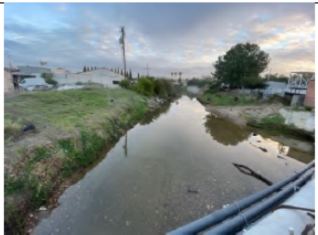
Photo Point 2 – Post-maintenance: Looking northeast above channel from National Ave. bridge at maintenance area following sediment and vegetation removal (January 17, 2022).
