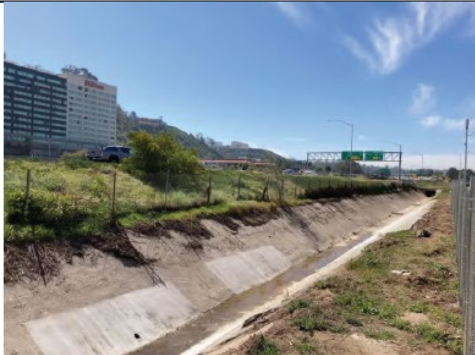
Post-Maintenance Photo Point 7: Looking northwest from the southern end of Camino del Rio 1 – vegetation shown to be removed from channel (3/2/2022).
