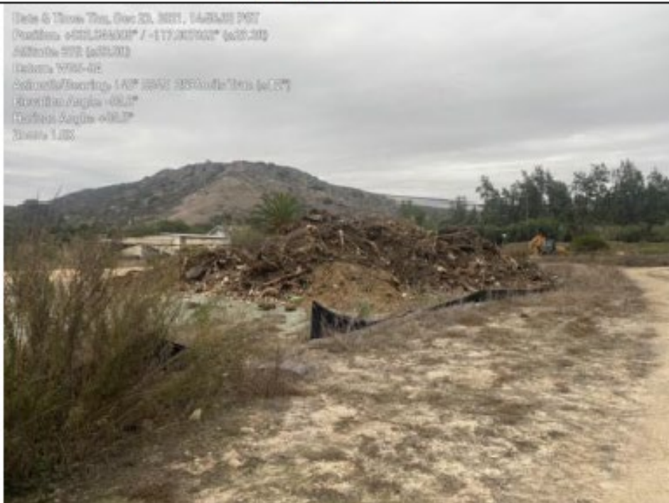
Photo 4: Stockpile in staging area with silt fence and fiber rolls installed (12/23/2021).
