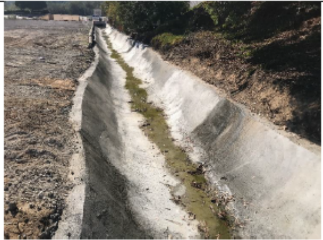
Post-Maintenance - Photo Point 5: Post-maintenance photo facing southwest from the developed concrete-lined channel looking at the cleared and repaired concrete lining in the Industrial 2 channel. Fence in pre-maintenance photo in developed area will be re-installed at a later date.
