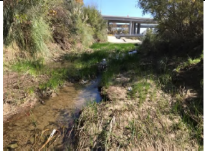
Roselle Post-Maintenance - Photo 7: View of Roselle 1 (earthen channel), looking south. Maintenance activities shown to be complete
