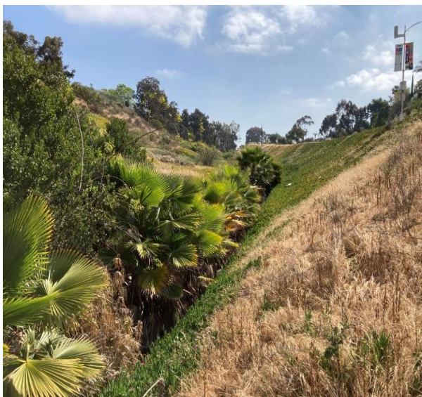
Photo 15: Facing upstream of the Washington 2 segment pre-maintenance. Taken June 1, 2021.
