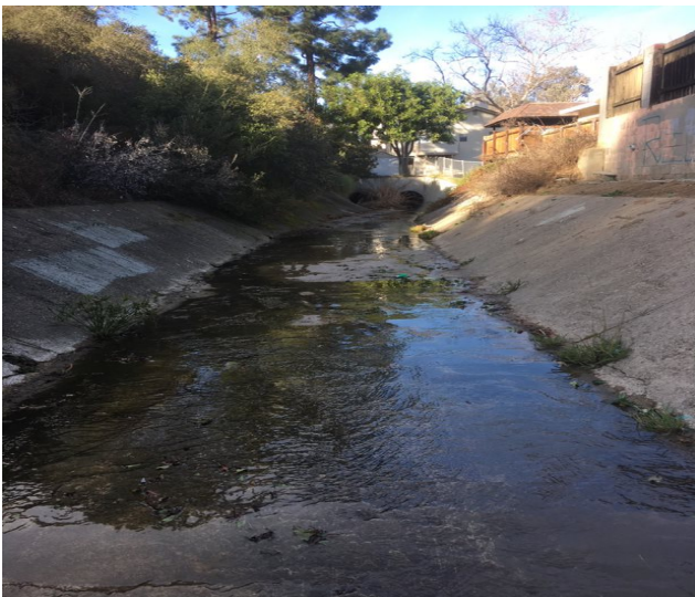
Photo 7: Facing downstream pre-maintenance. Taken January 28, 2021.
