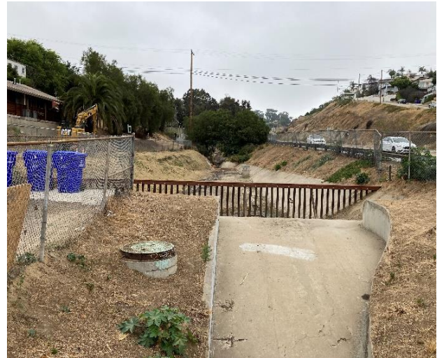
Photo 14: At the downstream section of the Washington 1 segment post-maintenance. Taken June 28, 2021.
