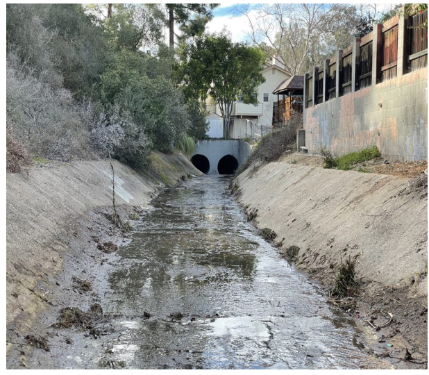
Photo 8: Facing downstream post-maintenance. Taken January 28, 2021.
