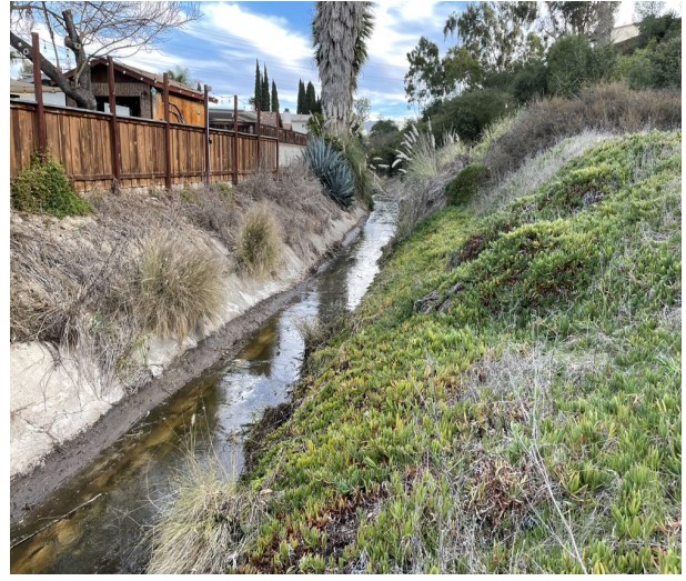
Photo 6: Chateau 1 Channel facing downstream post-maintenance. Taken January 28, 2021.
