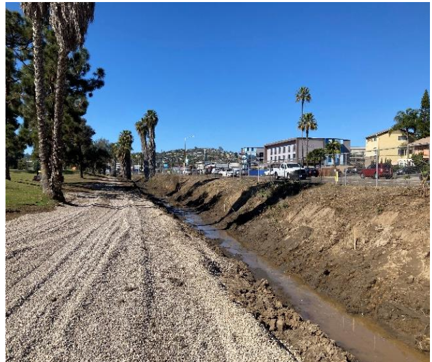
Photo 2: Facing upstream of the Mission Bay Drive-1 Channel following vegetation and sediment removal. Taken February 6, 2021.
