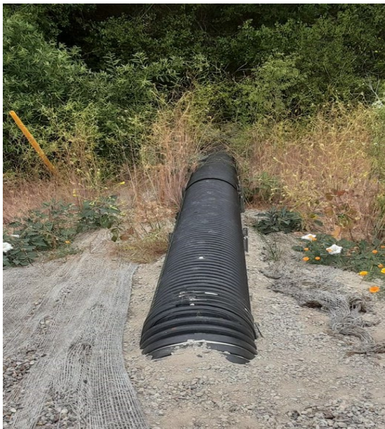
Photo 19: Facing downhill showing above-ground section of new HDPE installed. Taken May 20, 2021.
