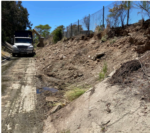
Photo 11: Facing downstream of the Mission Gorge 4 channel segment prior to concrete repairs showing the degraded concrete bank. Taken June 8, 2021.
