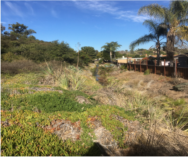
Photo 5: Chateau 1 Channel facing upstream pre-maintenance. Taken January 28, 2021.
