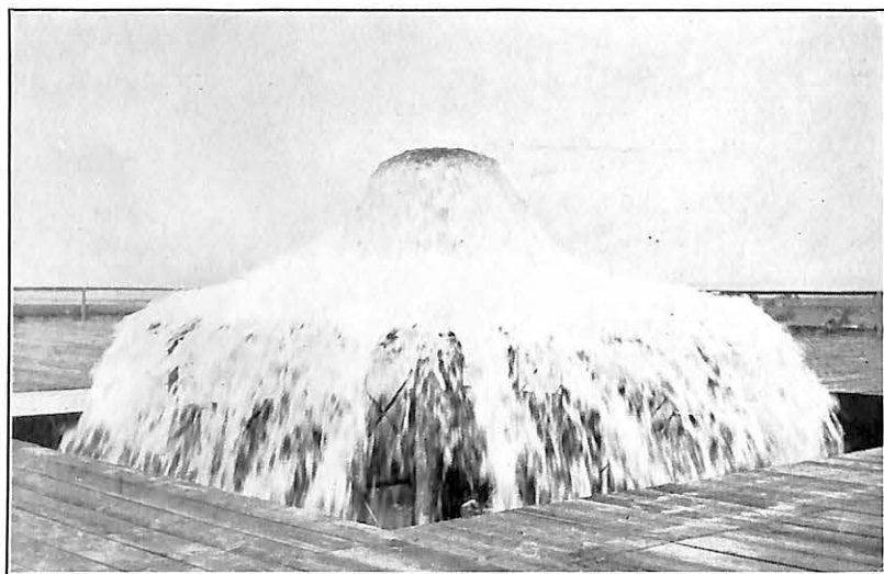
METHOD OF AERATING WATER RECEIVED FROM PIPE LINE BEFORE IT ENTERS UNIVERSITY HEIGHTS RESERVOIR
