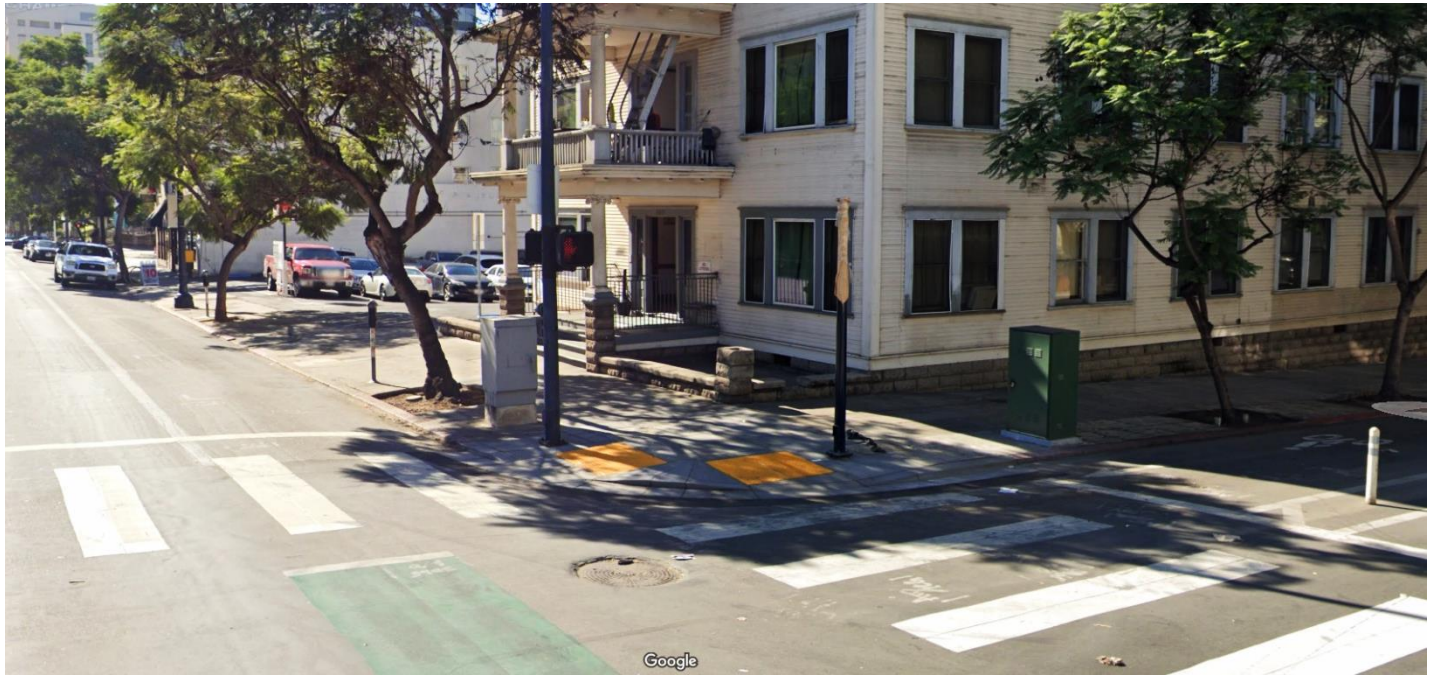
Example 04 – Dual Curb Ramps at a signalized intersection (Beech St. @ 1 st Ave.)
