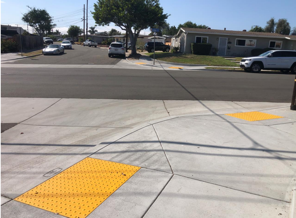
Example 06 – Dual Curb Ramps at a corner (Limerick Ave.@ Triana St.)
