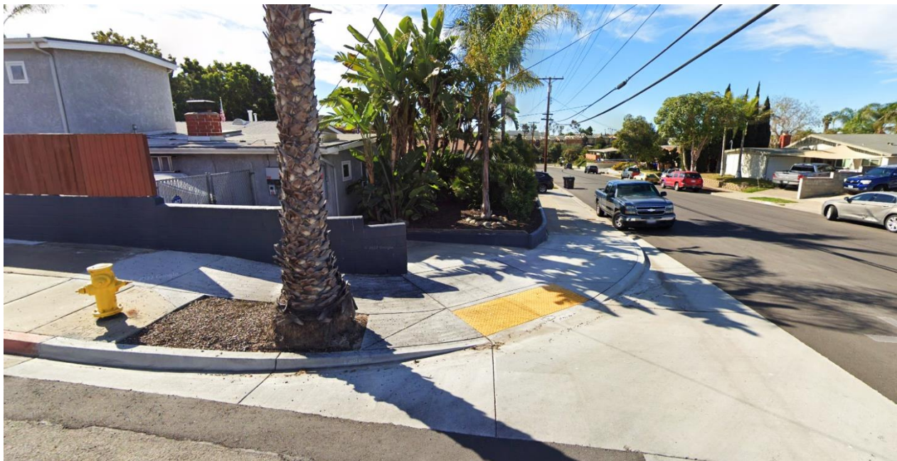
Example 07 – Single-wide (modified) curb ramp at a corner (Lyric Ln. @ Bowden Ave.)
