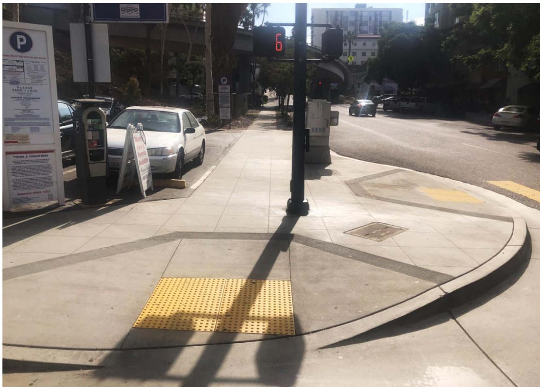
Example 03 – Dual curb ramps at a curb extension (W. Cedar St. @ Front Ave.)
