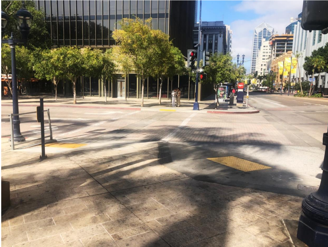
Example 02 – Dual curb ramps at a signalized intersection (Broadway Ave. @ 3 rd Ave.)
