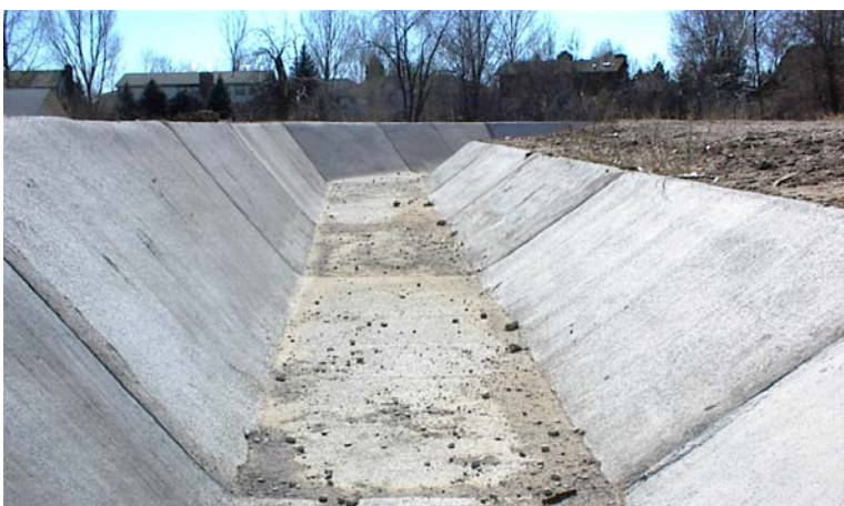
Figure 7-4. Example of Concrete-Lined Channel
