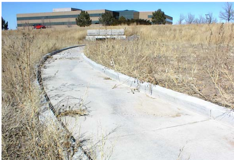
Figure 7-7. Example of Concrete Trickle Channel
