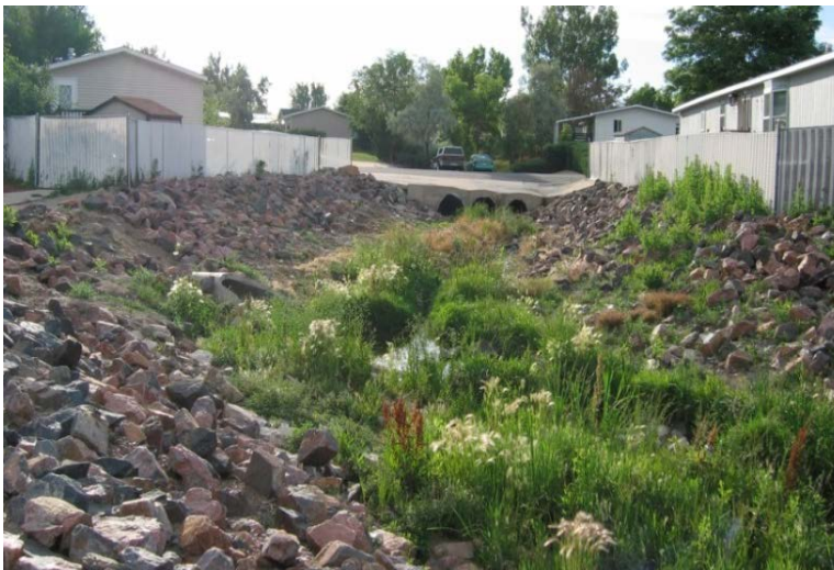
Figure 7-3. Example of Riprap-Lined Channel
