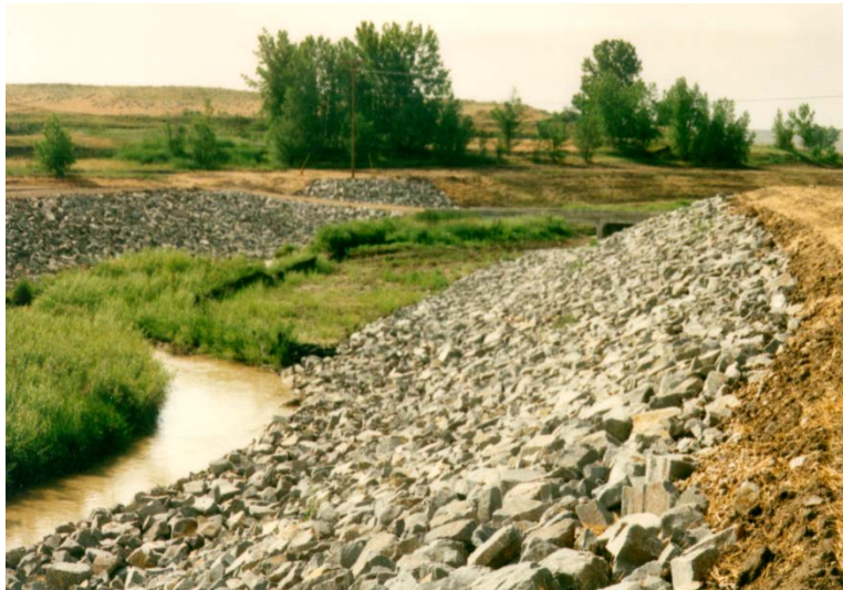
Figure 7-6. Example of Bank-Lined Channel
