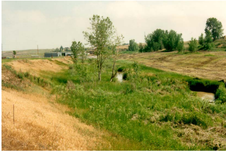
Figure 7-2. Example of a Wetland-Bottom Channel
