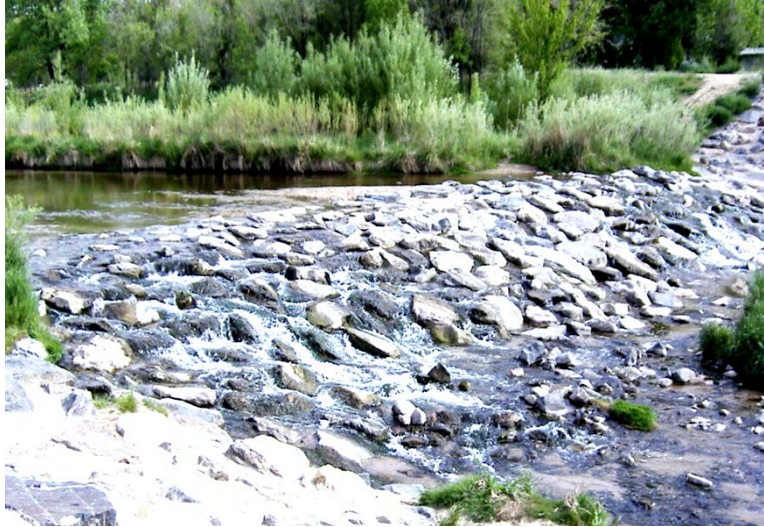
Figure 7-18. Example of Sloping Grouted Boulder Drop Structure
