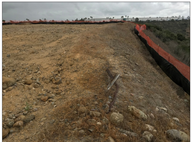
Photo 6: View of west side of restoration area facing south (5/2/2018)
