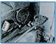
the emergency button at the top near the cabin lighting fixture and a 2kg emergency fire extinguisher.
